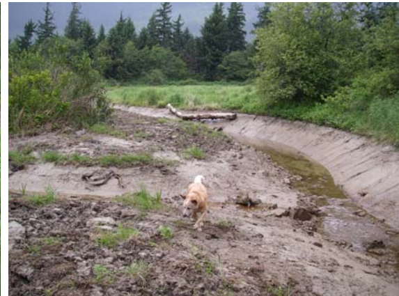
New channel facing west
