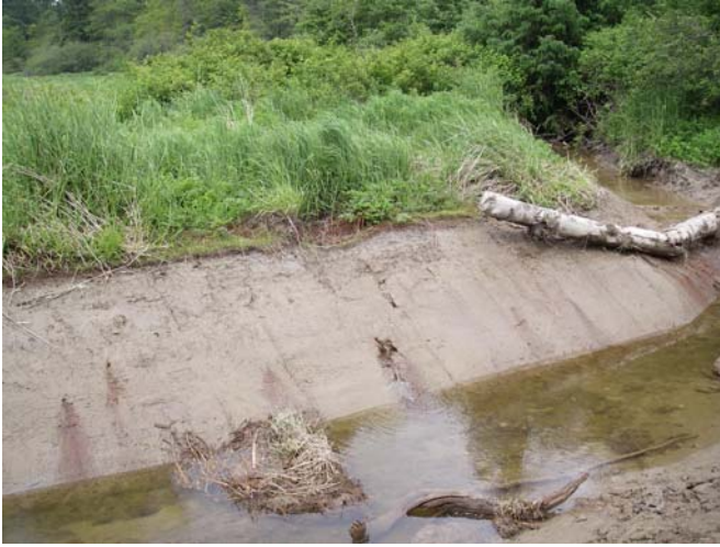
Notice piping (submerged channels) that allow seepage (right photo is close up)
