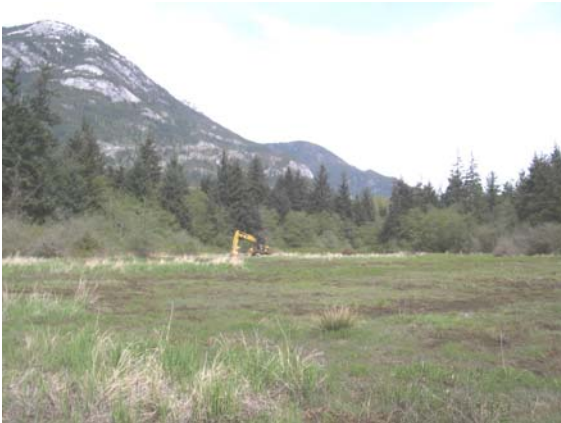
Getting started (north end of Site “A”)
