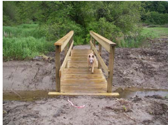
new bridge (with newly connected channel)
