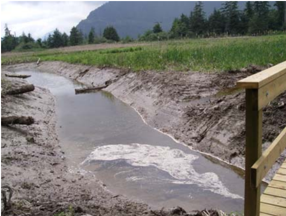
Downstream of new bridge – note how channel now connects with phase I
