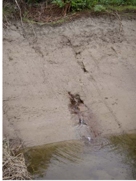
Notice piping (submerged channels) that allow seepage (right photo is close up)
