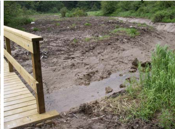
Upstream of new bridge
