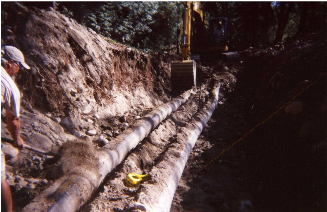
Figure 10 River Springs Oxbow Lake Intake Pipe Regrading
