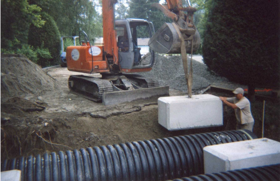
Figure 9 River Springs Oxbow Lake Outfall Pipe Replacement and Lock Blocks
