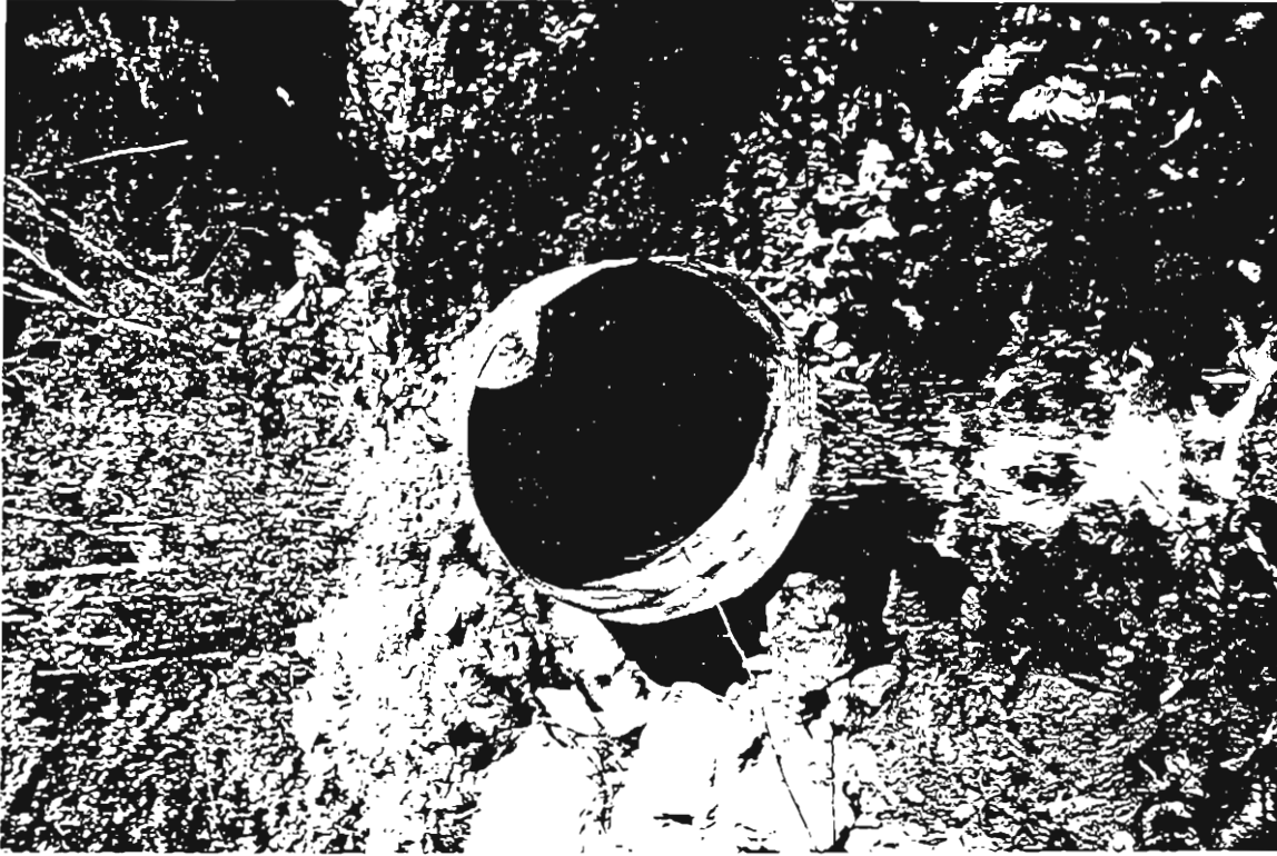
Figure 34. Recent culvert installation on Tributary 20, 115m upstream of Downton Lake.
