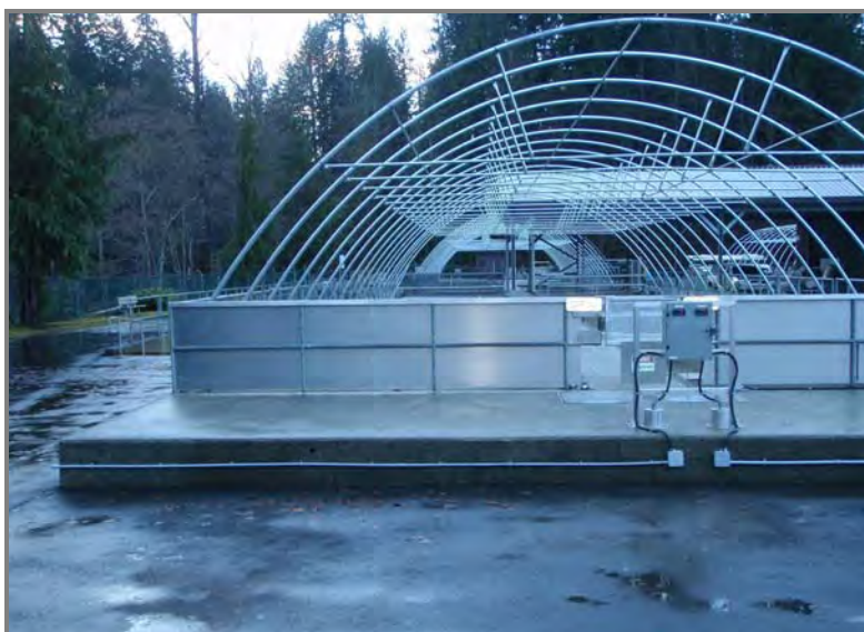
Figure 2. Upper end of the Puntledge Hatchery raceway that would accommodate the chilled holding tank. The chiller unit would be located on the adjacent concrete pad.
