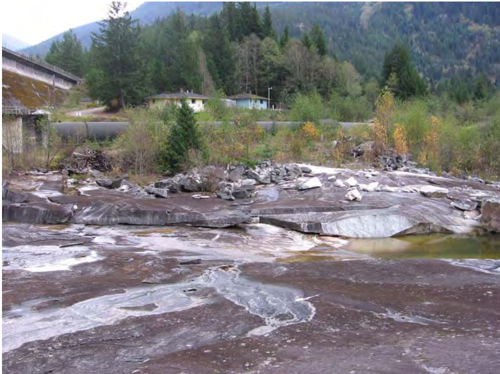
Photo 16: Cross channel view below spillway from right bank.
