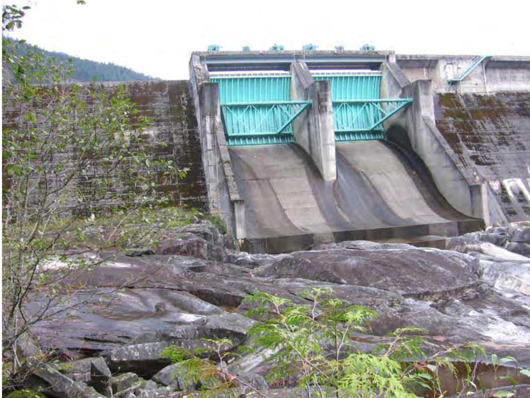
Photo 15: Upstream view of spillway from right bank.
