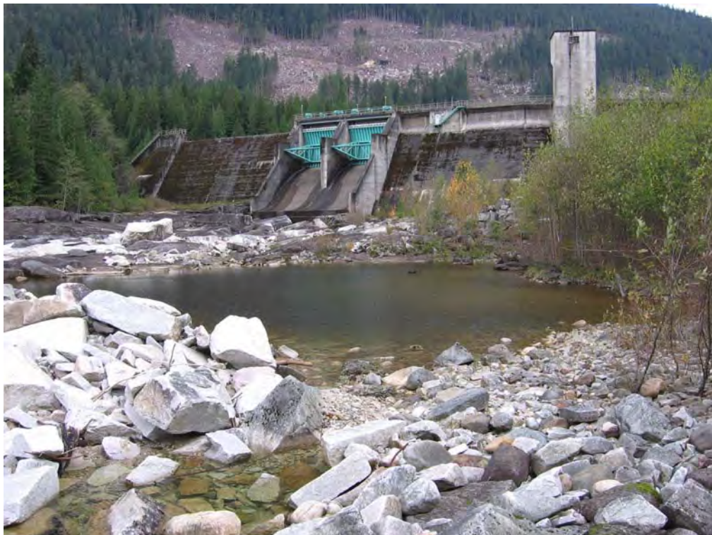
Photo 12: Upstream view from left bank above Interfor bridge.
