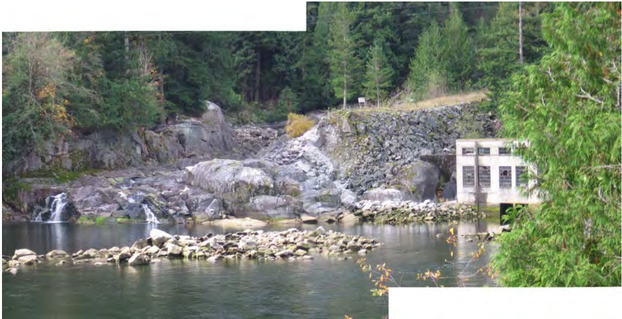
Photos 1 & 2: View across Salmon Inlet of Clowhom River spillway and powerhouse.
