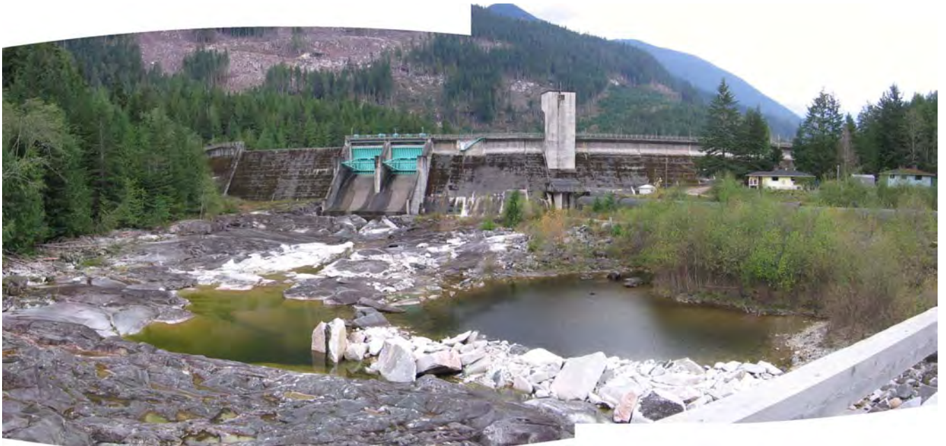
Photos 13 & 14: Upstream view of bypass reach from bridge.
