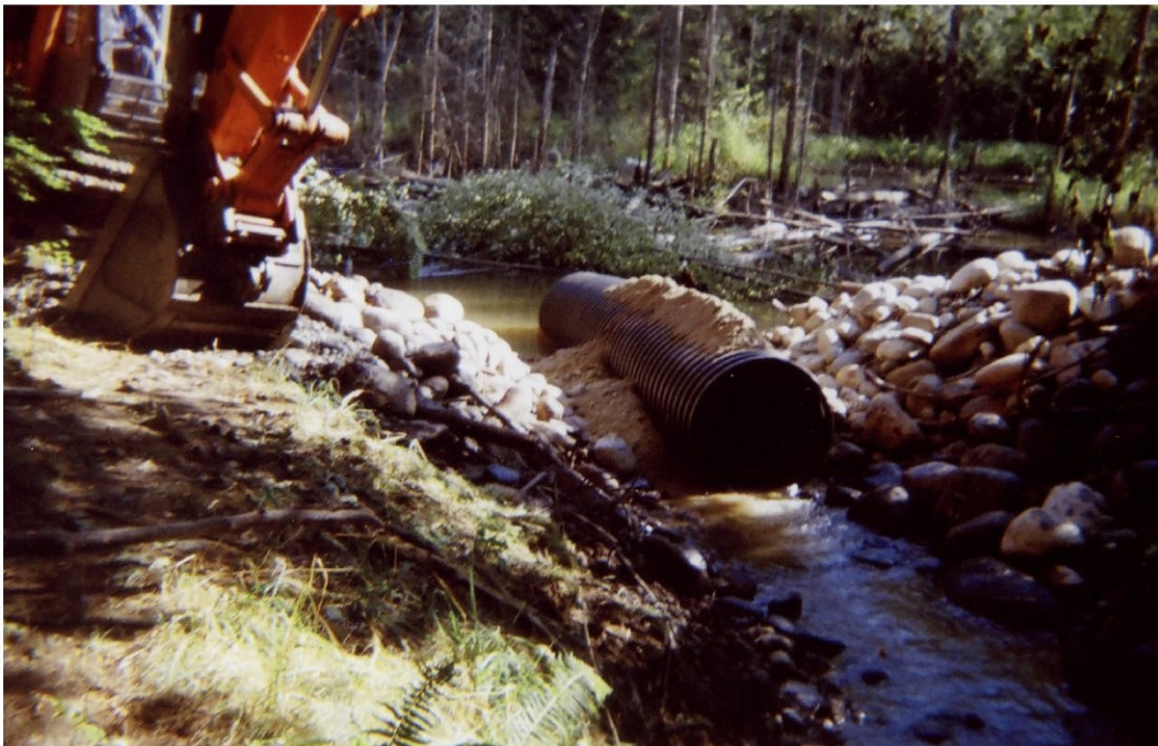
Figure 8 Oxbow Pond Beaver Bafflers Pipe Installation
