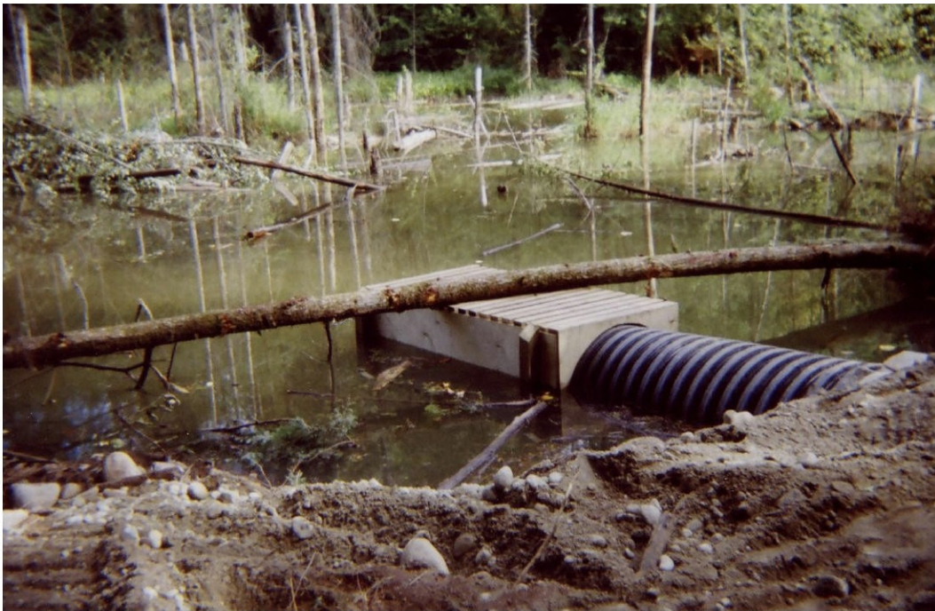
Figure 10 Oxbow Pond Beaver Baffle After
