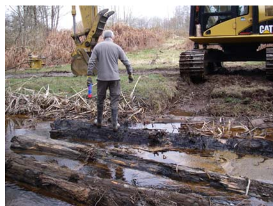
Access cordons across easternmost branch by Dentville (all access was removed at the end of the project)
