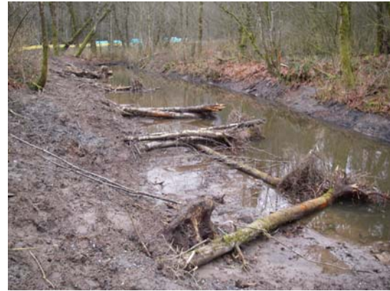
Clearing the site (the LWD to be used later as seen on right photo)
