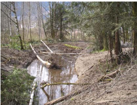
Tidal Slough after being deepened
