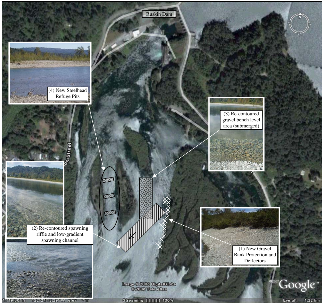
Figure 5. Final project results and locational map of (1) bank protection, (2) re-contoured spawning riffle/channel, (3) gravel bench, and (4) new steelhead refuge pits
