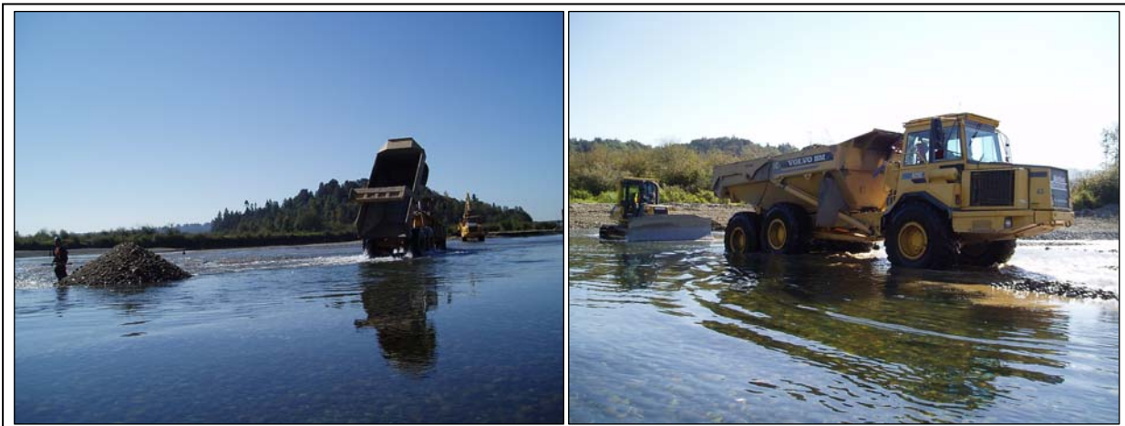
Figure 3. Project construction (September 2007)
