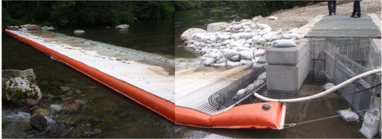
Figure 5: The newly constructed Allco fish trap, 2008.
