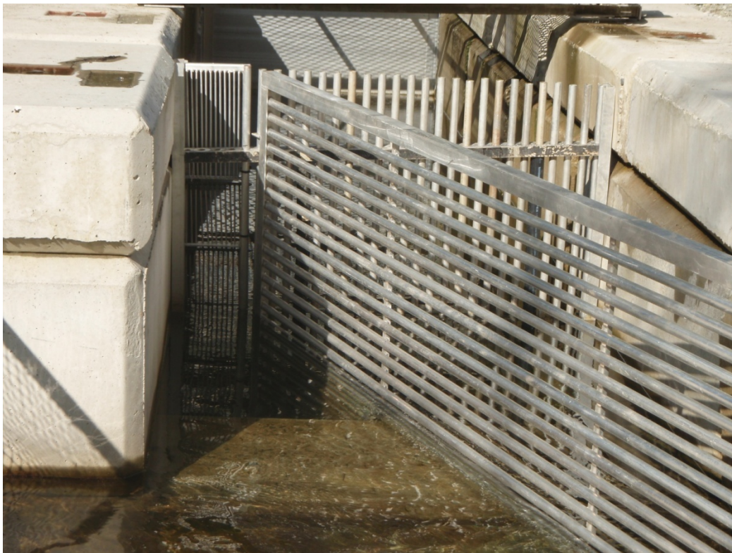
Figure 4: Finger-gate and entrance of the new trap, 2009.
