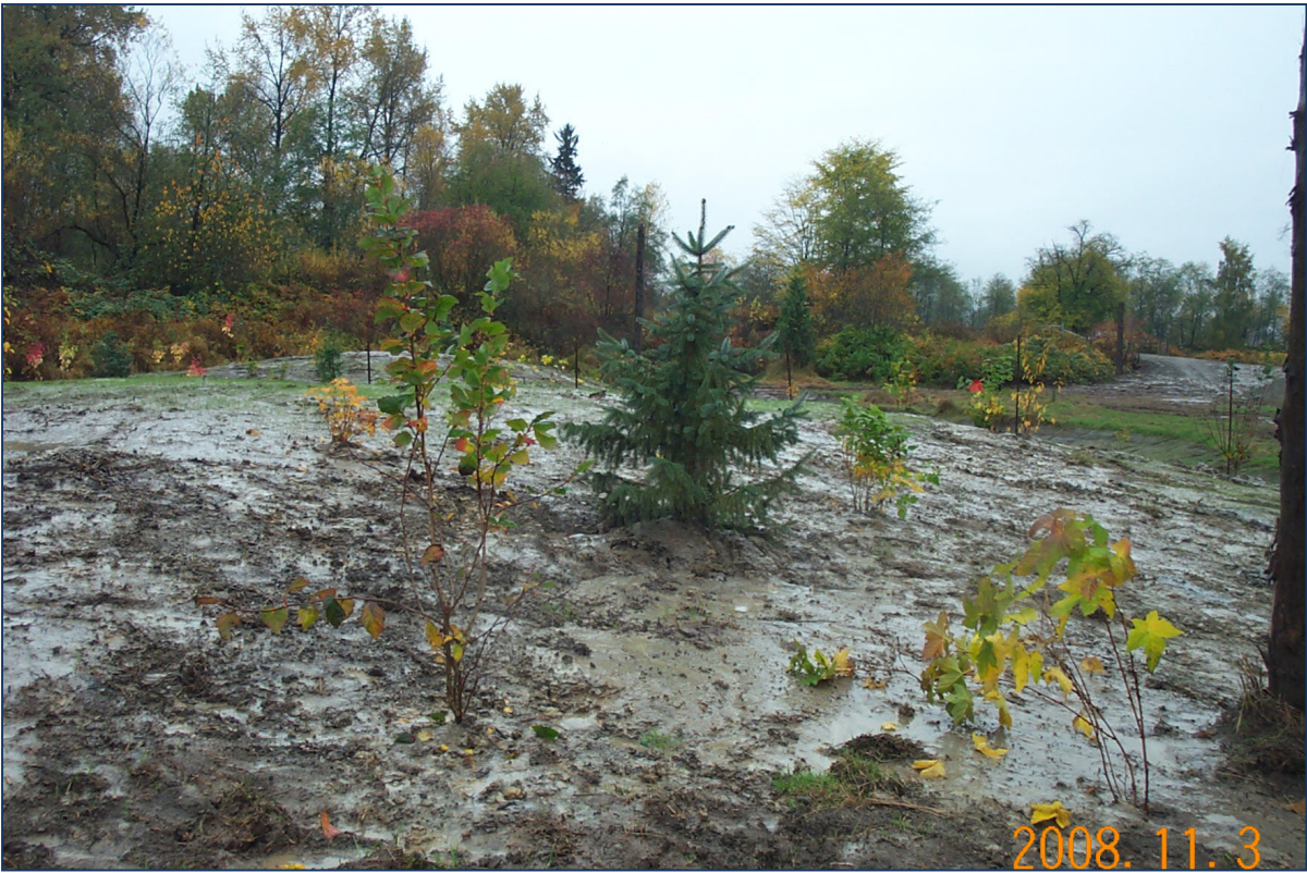
Figure 13 Construction –Large Specimen Planting
