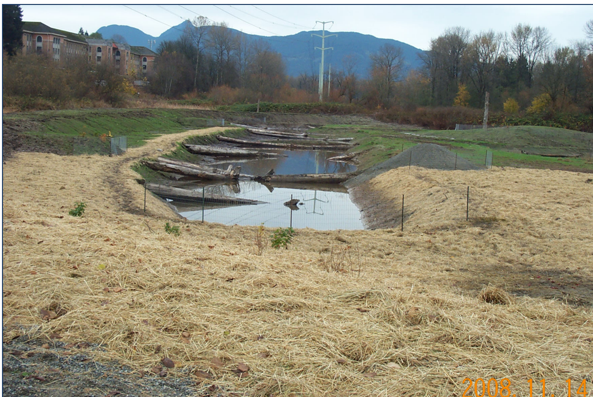
Figure 7 Project Site Week 8 Completion
