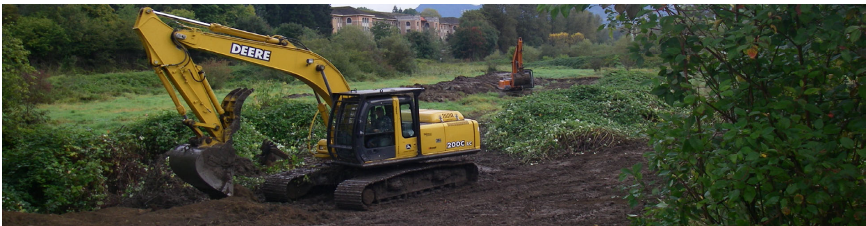
Figure 3 Large Tracked Machines on Site
