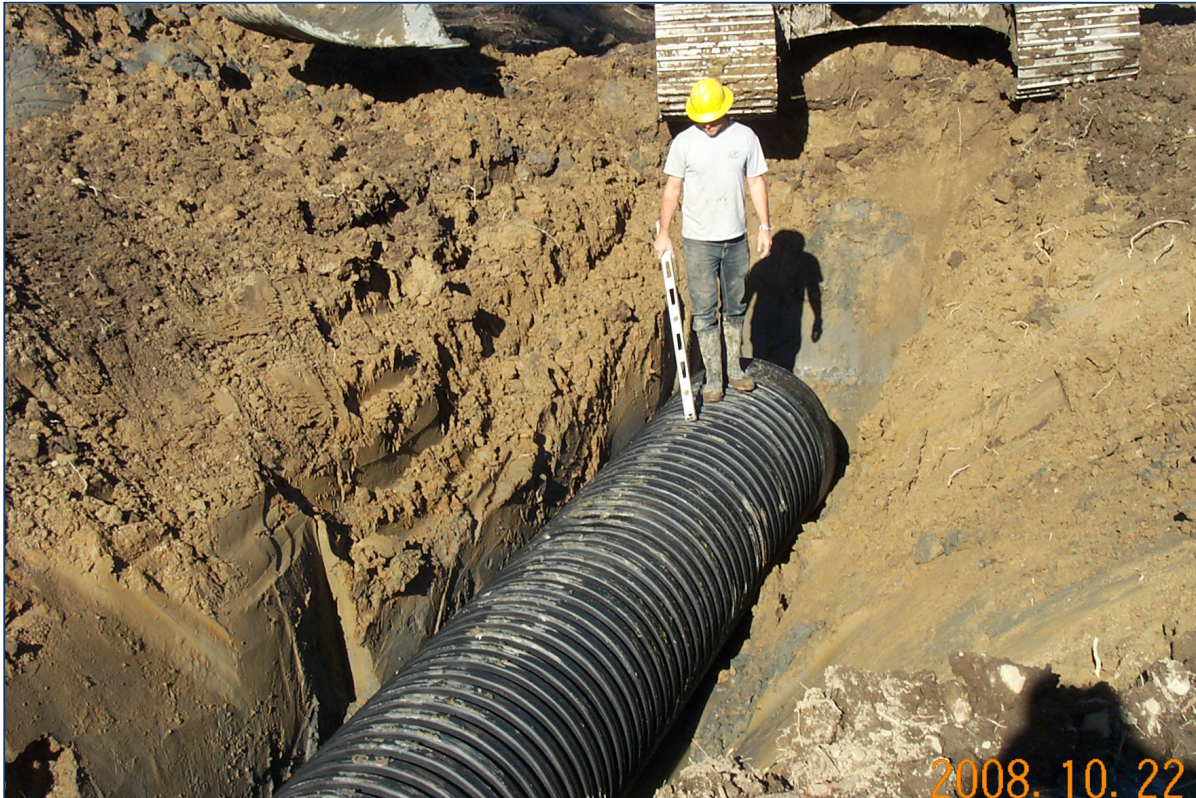
Figure 10 Construction – Installing Culverts
