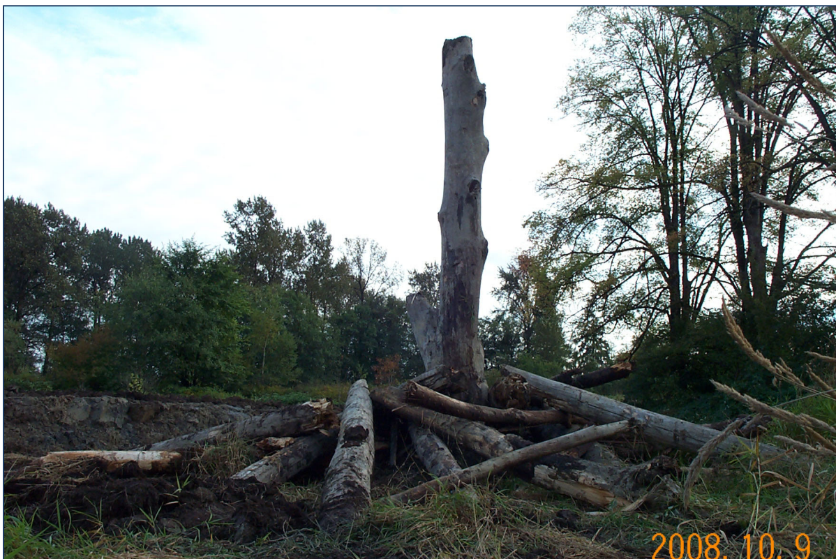
Figure 11 Construction – Installing Bird of Prey Perching Posts and Wildlife Woodpiles
