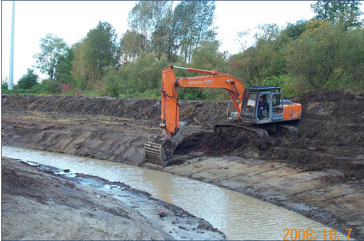
Figure 8 Construction - Main Channel
