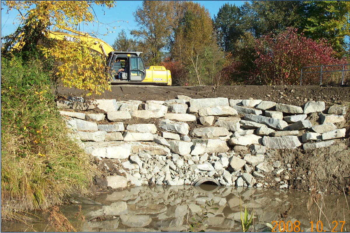
Figure 12 Construction – Completing South-facing Reptile and Amphibian Hibernacula
