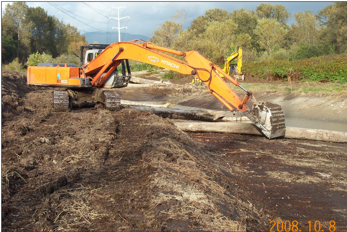
Figure 9 Construction – Keying in Large Woody Debris
