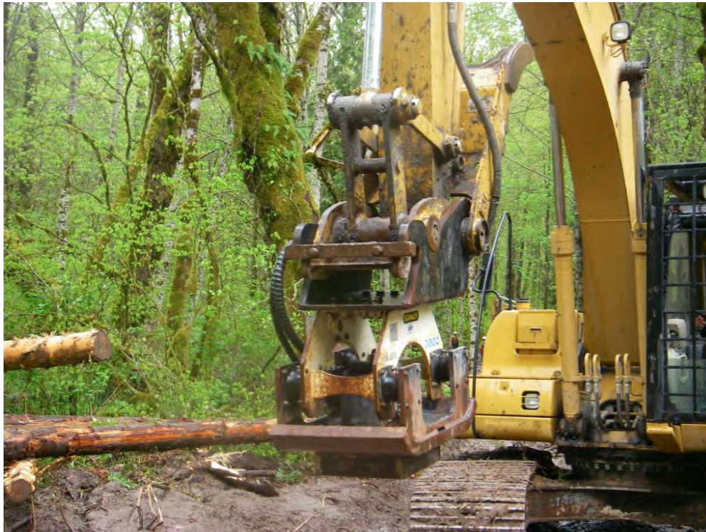
Photo 1. Vibratory Pile Driver attached to excavator (photo credit D. Harper, BCCF).
