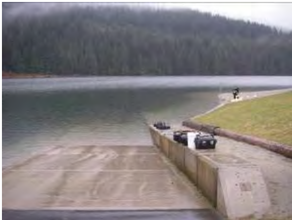
Preparing assembly site for the delivery on the dock section.
