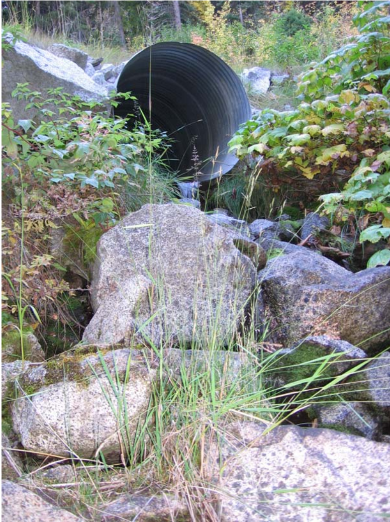
Photo 032 Outlet upstream photo
