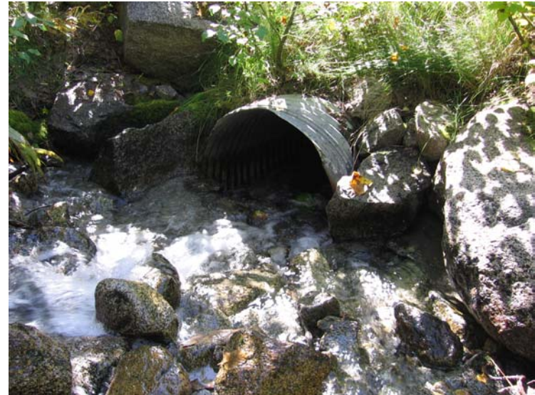
Photo 038 Inlet downstream photo
