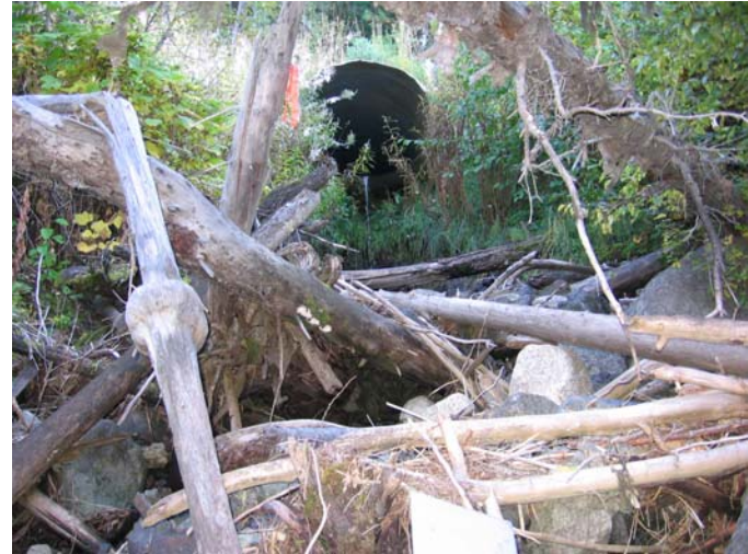
Photo 008 Outlet upstream photo
