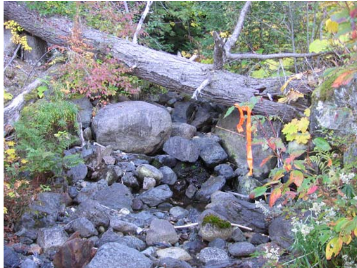
Photo 007 Inlet downstream photo
