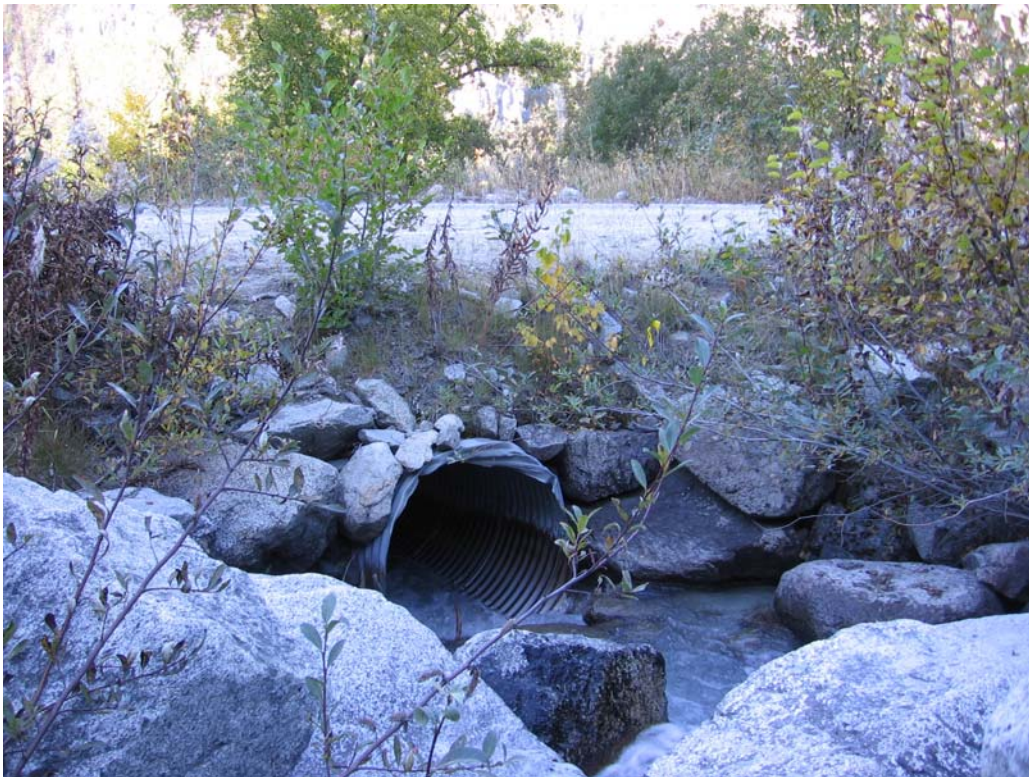
Photo 040 Inlet downstream photo
