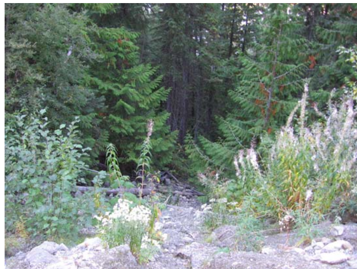
Photo 012 Downstream of outfall – no channel.
