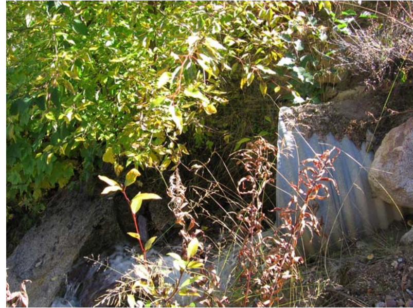
Photo 024 WP 020 View of culvert from side showing outfall drop.
