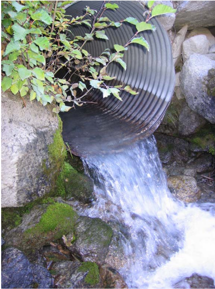
Photo 041 Outfall upstream photo
