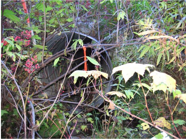
Photo 030 Inlet downstream photo
