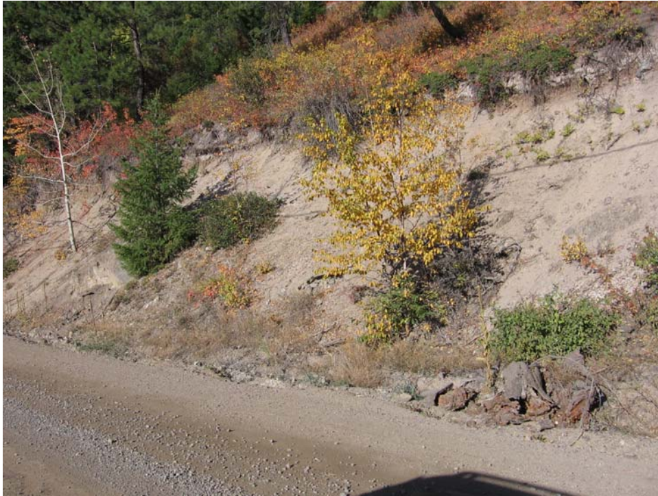
Photo 014 View southwest along Gun Creek FSR.
