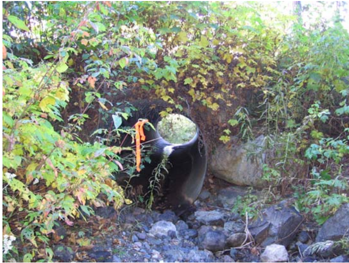
Photo 006 Inlet upstream photo
