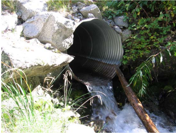
Photo 035 Outfall upstream photo
