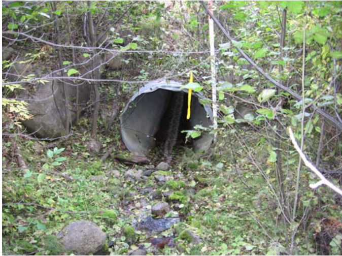
Photo 001 Downstream view of inlet
