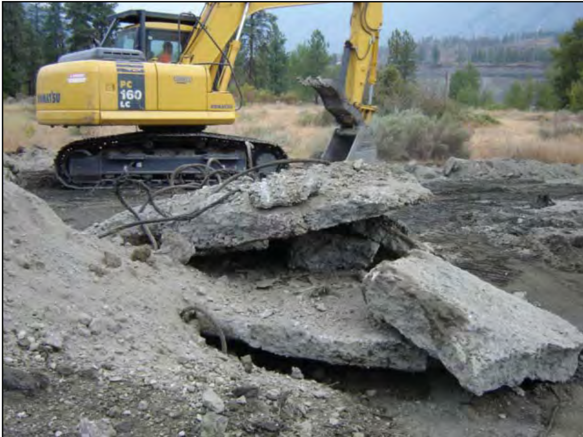
Fig 41 Concrete slabs being uncovered
