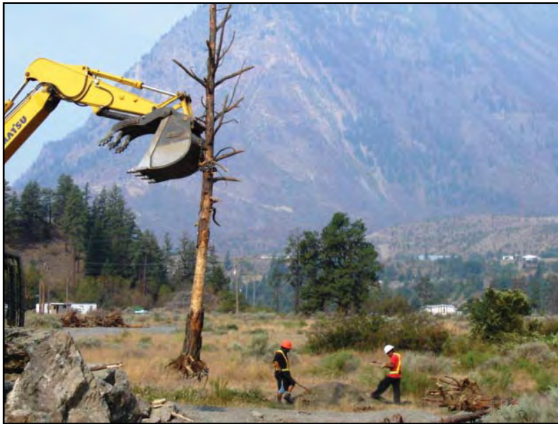
Fig 45 - 47 Snag being lifted for planting, soil being backfilled and installed snag Polygon 05
