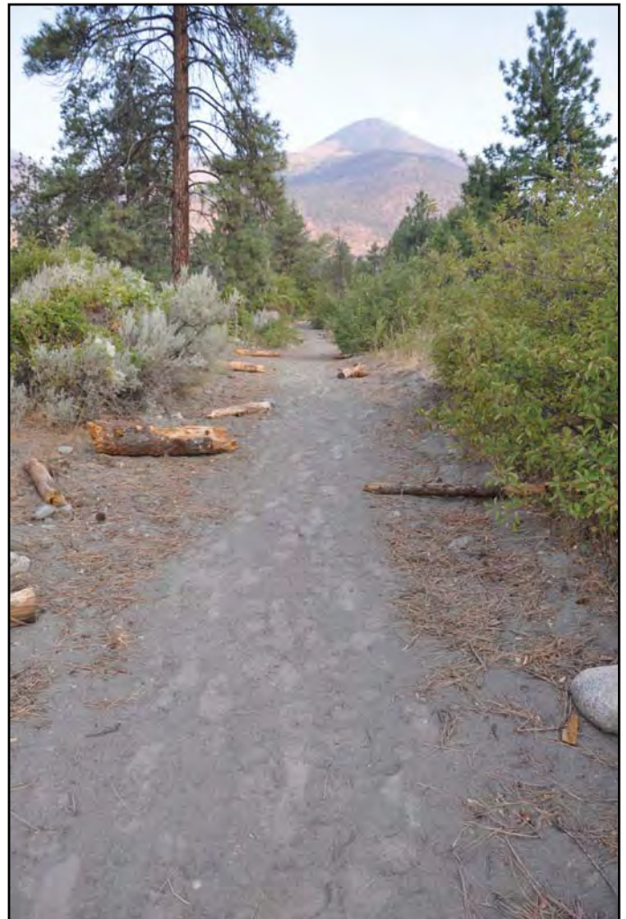
Fig 36 Same road after work July 2009
