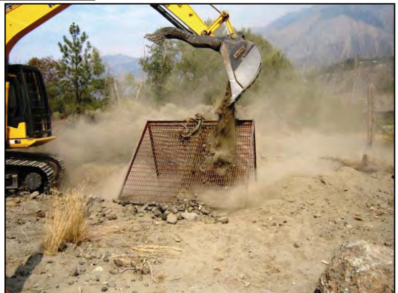
Fig 39 Smaller chunks of asphalt being screened out of soil
