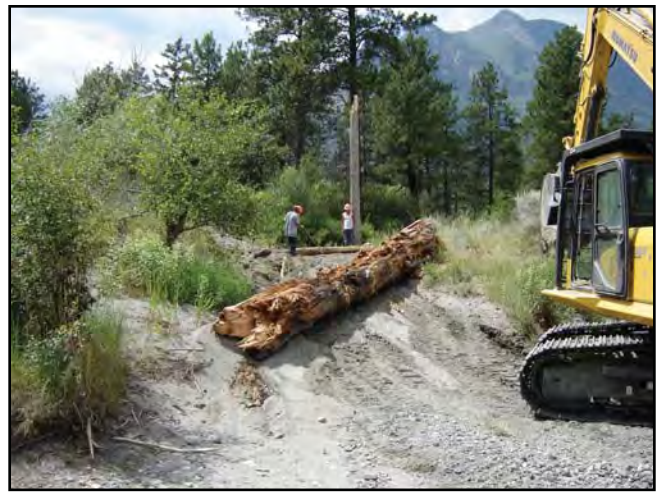
Fig 19 Road deactivation at north end of site 2008
