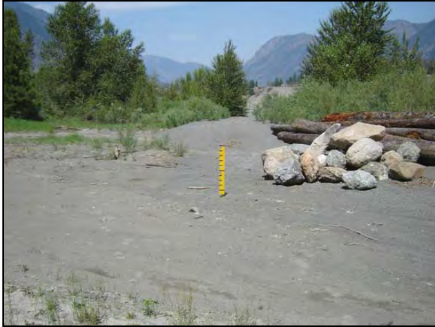
Fig 134 PP04 North BEFORE road closures July 02, 2008
