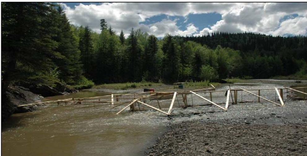
Fish fence/trap structure installed on Johnson Creek to monitor use and spawning success of rainbow trout.
