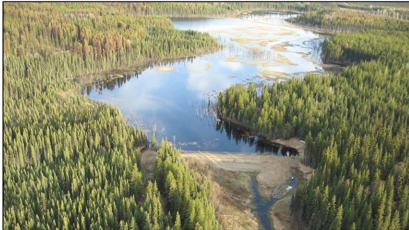
Water-control structure (earthen dam with variable-crest drop inlet) and wetland at Rocky Marsh (25 ha).
