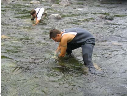
Figure 4a and 4b. First Nations and BCCF crews securing pollock filled burlap bags to the bottom of the river using large cobbles.
