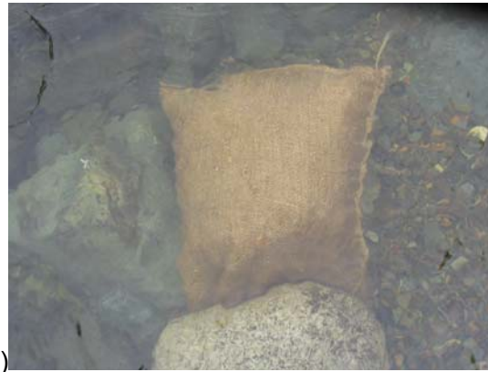
Figure 4a and 4b. First Nations and BCCF crews securing pollock filled burlap bags to the bottom of the river using large cobbles.
