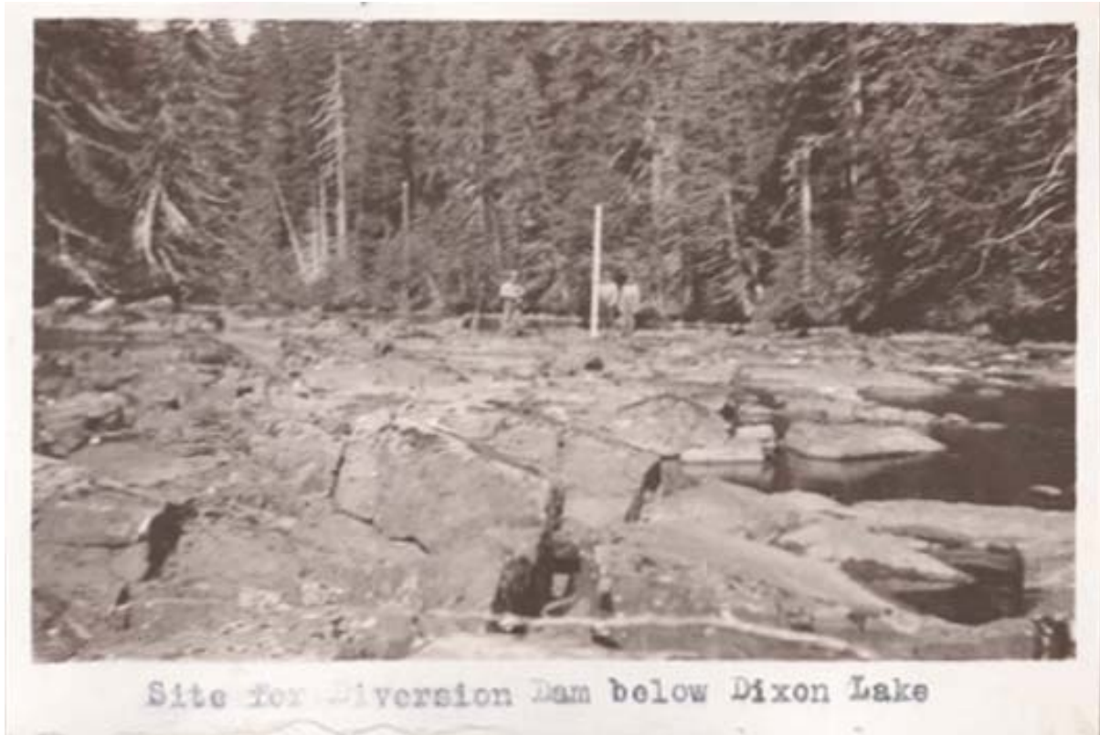
Figure 35. Potential site for a diversion dam below Dickson Lake (1922).
