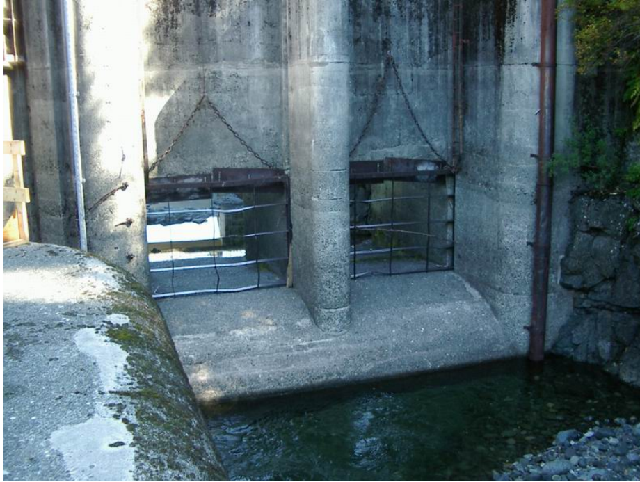
Figure 5. Upstream entrance to the diversion canal, looking downstream. Mainstem discharge ( 1.7\text{m}^3/\text{sec} in this photo) all carried through undersluice (1m open) to the left of photo. Shows relative sill height of canal entrance and trash rack on canal.
