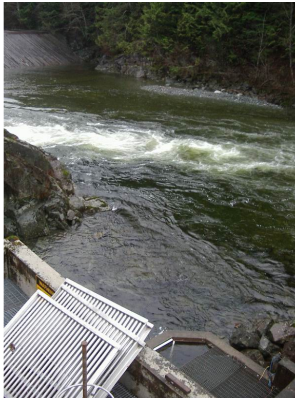
Figure 25. View of entrance to Salmon River fishway with mainstem in background. Screen is off lowest cell of fishway, where Coho could have bypassed resistivity counter both up and down.
