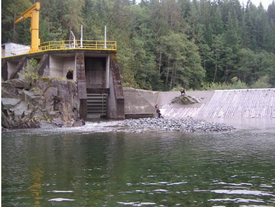
Figure 21. Salmon River diversion structure looking upstream - undersluice gate open to 0.9m September 24 2008, mainstem flow less than 1\text{m}^3/\text{sec} . All of the river flow is passing through the undersluice.
