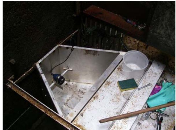
Photo 4. Camera tunnel installation in the Comox Dam fishway after cleaning, February 20, 2008.
