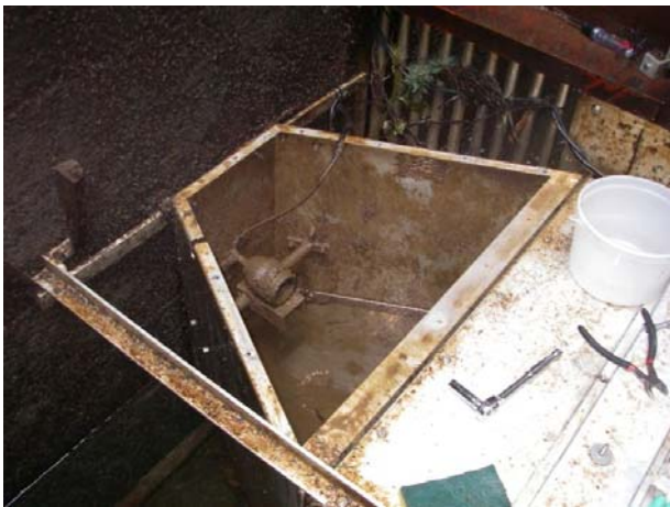
Photo 2. Camera tunnel installation in the Comox Dam fishway before cleaning, February 20, 2008.
