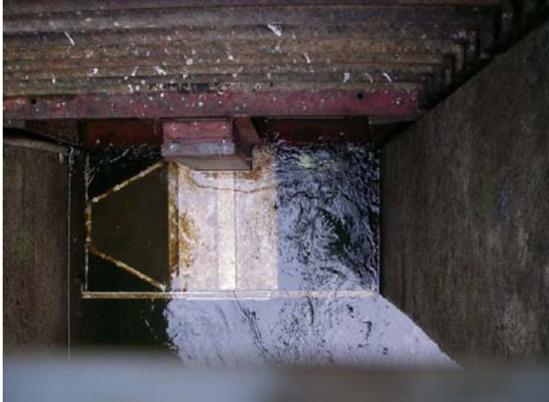
Photo 1. View of the camera tunnel from the top of the Comox dam fishway during low lake elevations (131.2 m), February 20, 2008.
