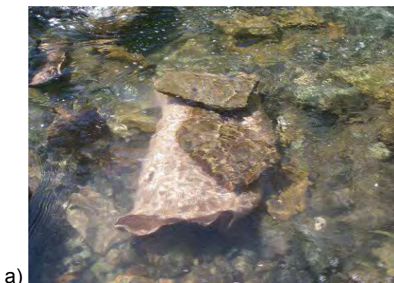
Figures 4a and 4b. Pollock filled burlap bags were secured to the bottom of the river using large cobbles.
