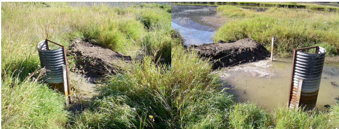
Figure 3 Earth dams built in front of outlets to pond 3 (right) and pond 4 (left).
