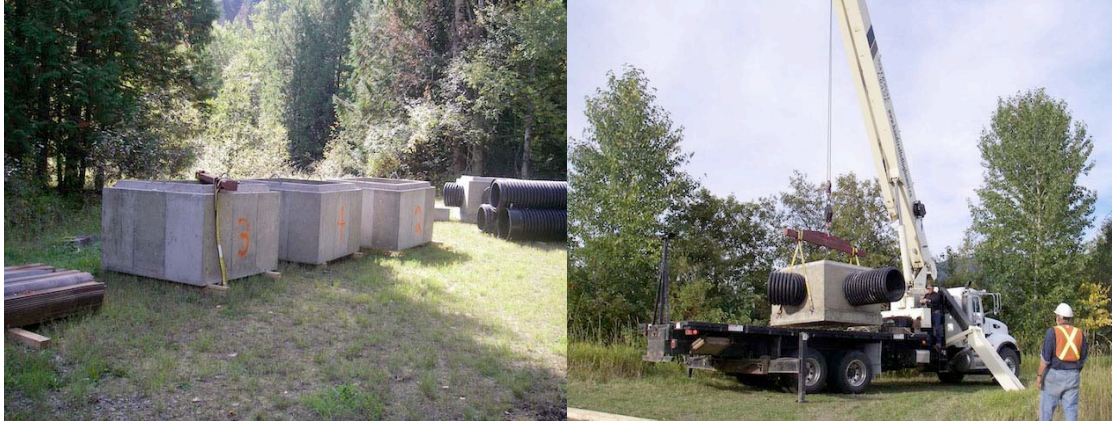
Figure 2 Water control parts (left) being unloaded at the project location (right).
