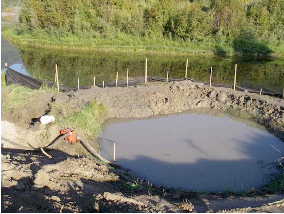
Figure 4 Earth dam on Kootenay River side and silt fence.
