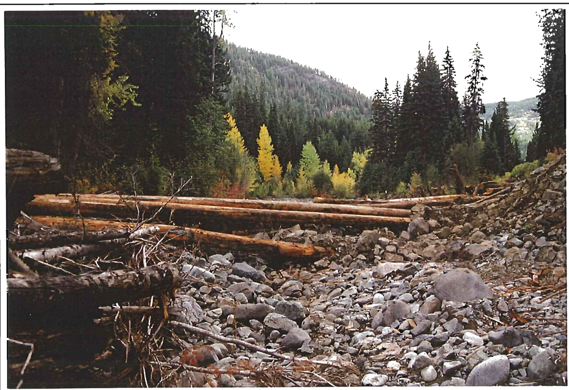
Photo 24: Granite Creek. View of Section 3 facing upstream at entrance to dry side channel. Post construction. (25 September 1997).
