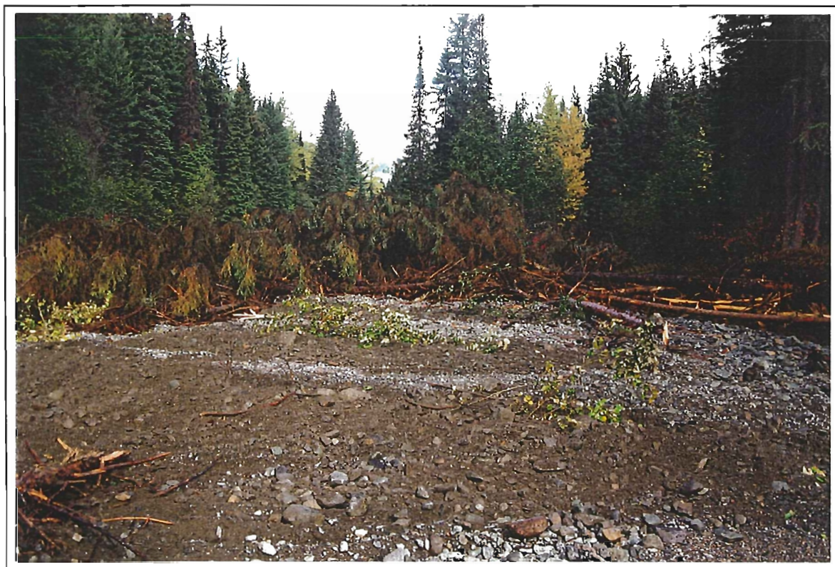
Photo 34: Granite Creek. View of Section 4. Post construction. Note: Nursetrees planted in gravel/ sand bar. (26 September 1997).
