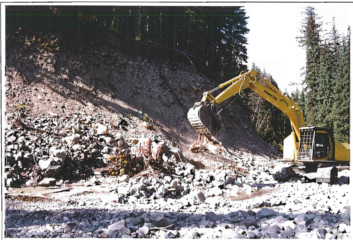
Photo 22: Granite Creek. View of Section 3. Mid construction.
