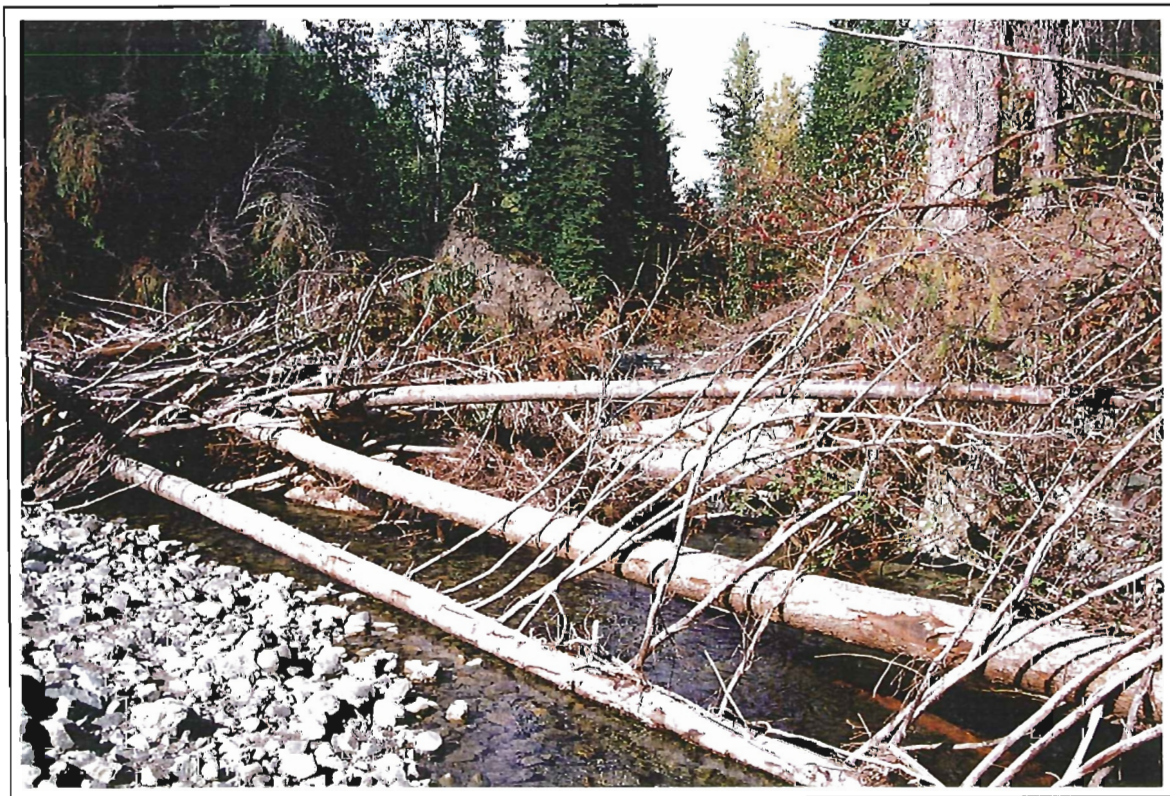
Photo 26: Granite Creek. View of Section 4 facing downstream. Pre-construction. Note: Logjam. (25 September 1997).
