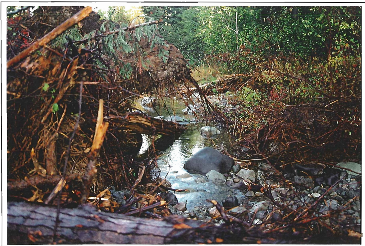
Photo 32: Granite Creek. View of Section 4. Channel flowing north. Post construction. Note: Flow decrease compared to pre-construction. (25 September 1997).
