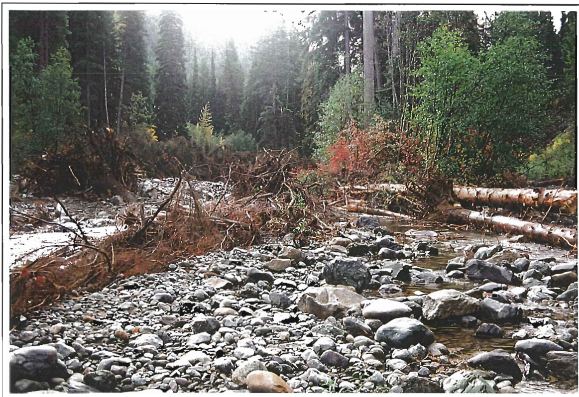
Photo 37: Granite Creek. View of Section 5 facing upstream. Post construction. Note: Large rootwad east bank, rootwad instream, stabilized west bank. (26 September 1997).
