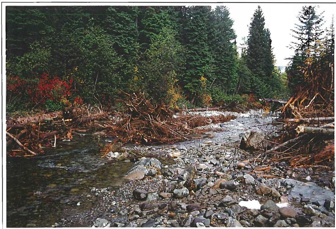
Photo 36: Granite Creek. View of Section 5 facing downstream. Post construction. Note: Rootwad instream, logs at west bank, debris at east bank. (26 September 1997).
