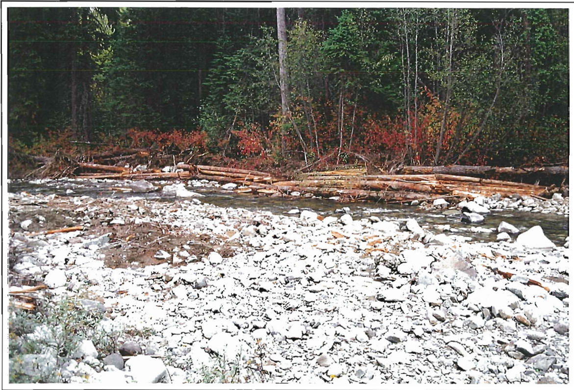
Photo 15: Granite Creek. View of Section 1 facing east bank. Post construction. (26 September 1997).
