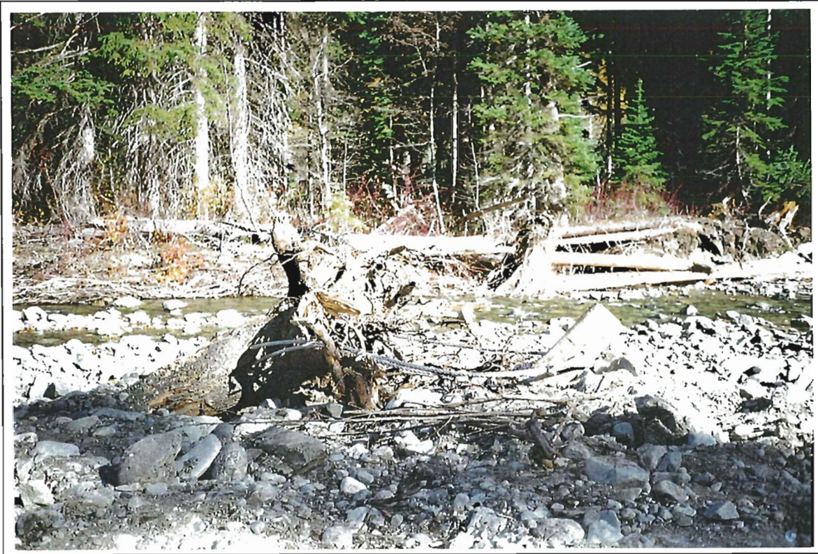
Photo 19: Granite Creek. View of Section 2. Post construction. Note: Rootwad cabled to deadman. (20 October 1997).
