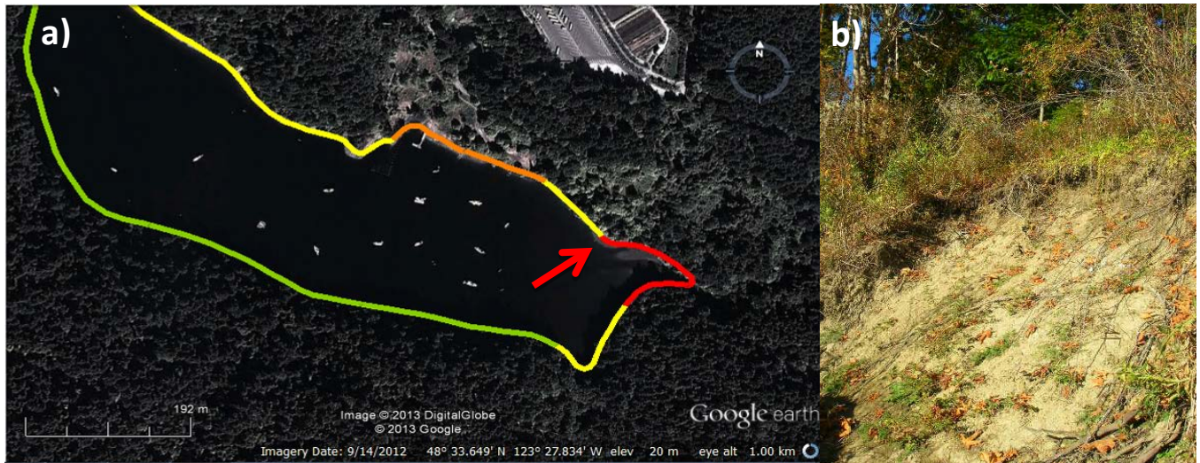
Figure 7. Estuary at Tod Inlet, Saanich Peninsula. a) Google Earth image with .kml file of shoreline sensitivity model; location of slump indicated with red arrow. b) Slump and scarp at shoreline were observed when the area was ground-truthed.
