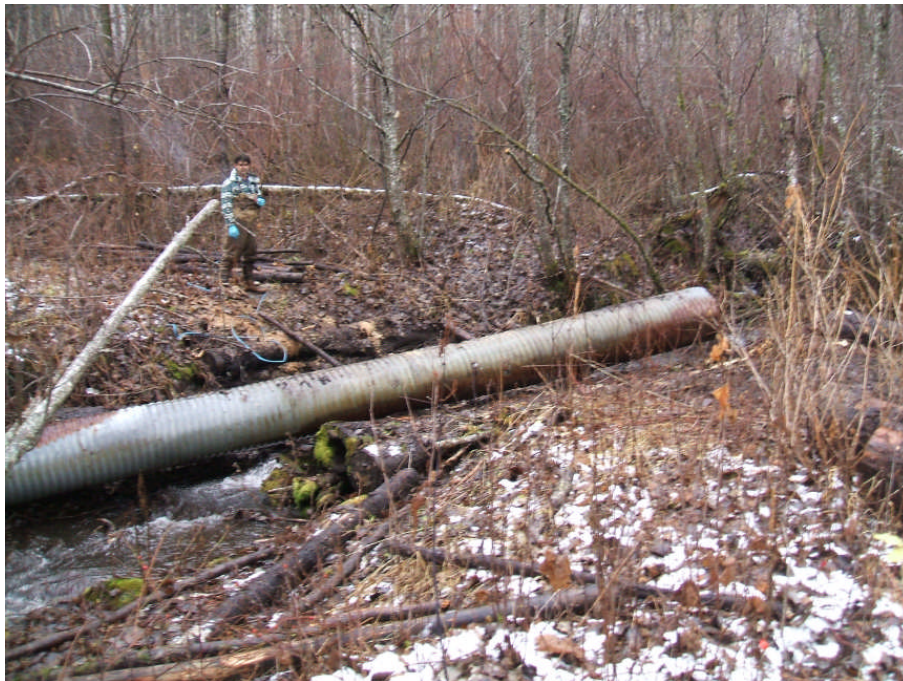
Photo 35: Removing culvert using ATV during deactivation at Site 48.
