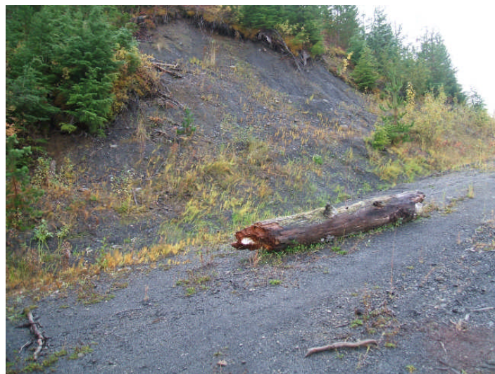
Photo 23: Site 35 – Mass wasting on left-road cutbank.
