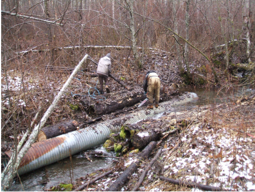
Photo 34: Removing logs over culvert during deactivation at Site 48.
