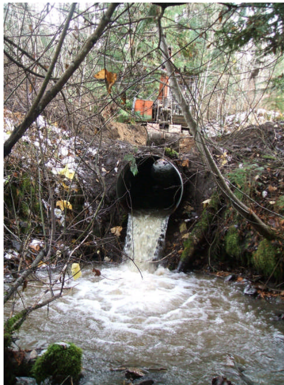
Photo 42: Removing fill material over Site 61 culvert outlet.
