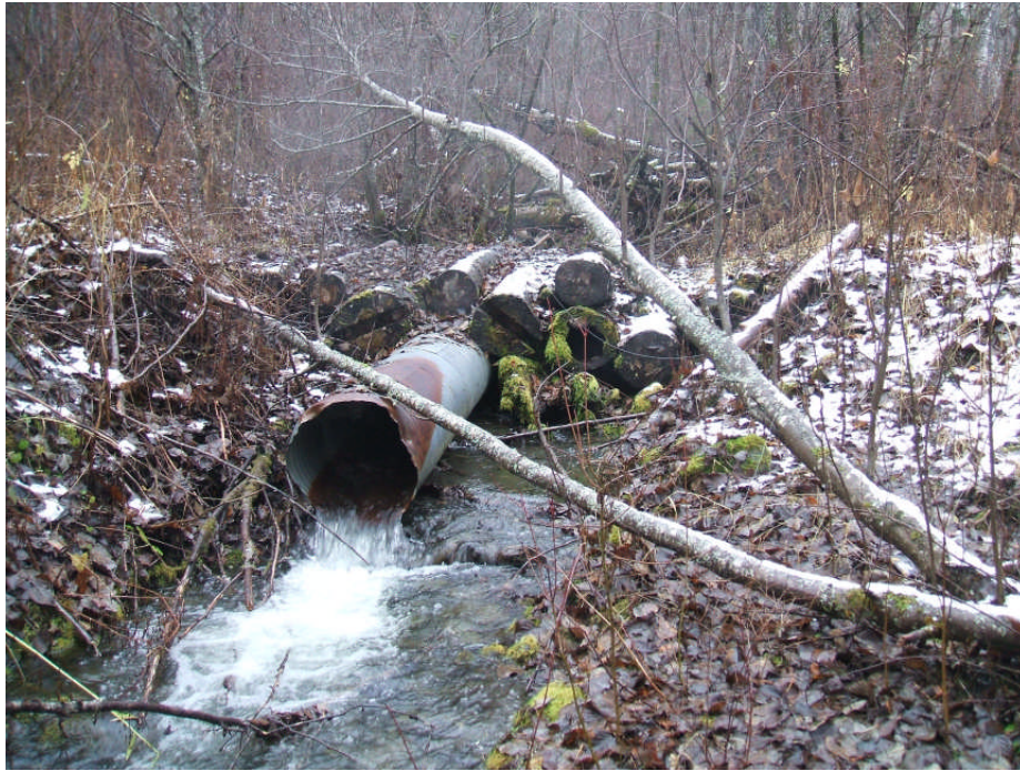
Photo 31: Log fjord and culvert outlet before deactivation.
