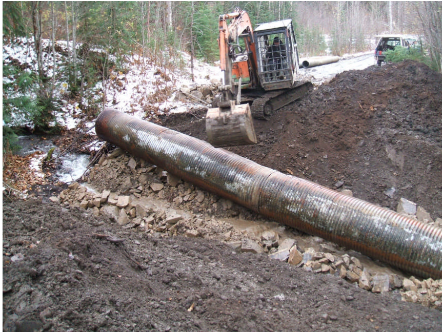
Photo 43: Removing culvert from streambed at Site 61.
