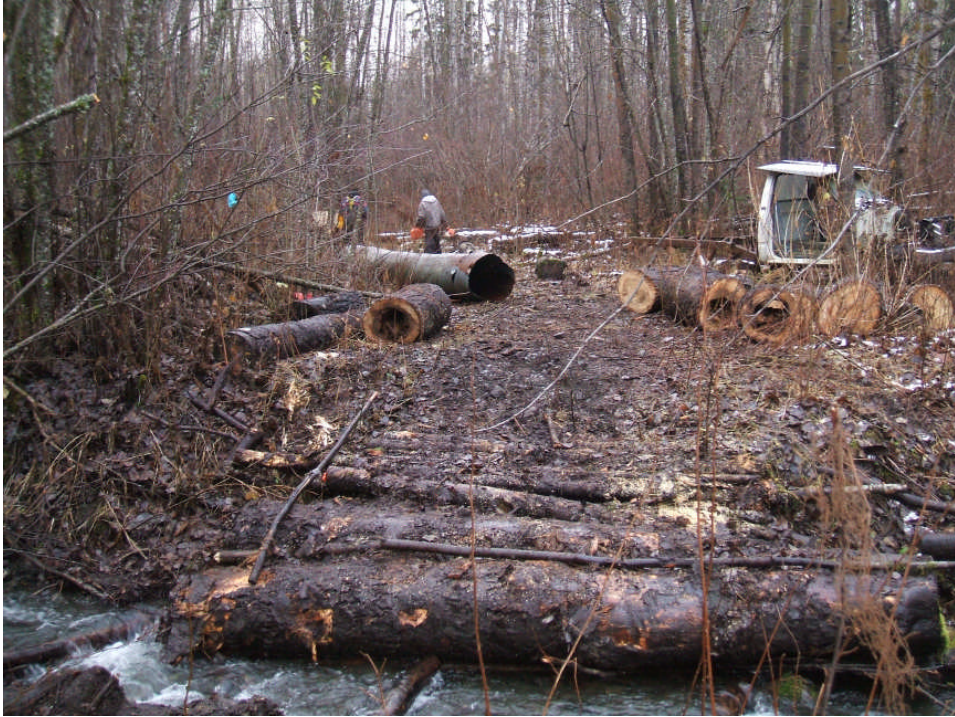
Photo 36: Culvert and logs removed from streambed and placed on left road surface.
