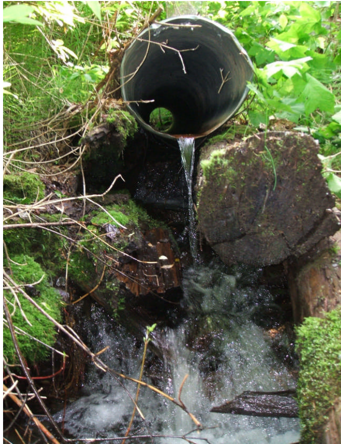
Photo 27: Site 14 culvert outlet prior to deactivation. Water was flowing mostly through the log corduroy in the underlying roadbed.
