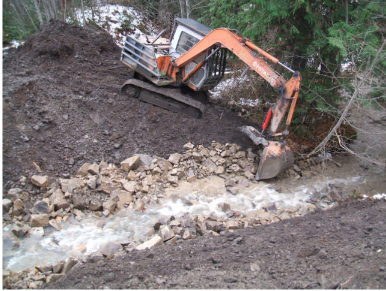
Photo 45: Final riprap placement along new channel at Site 61.
