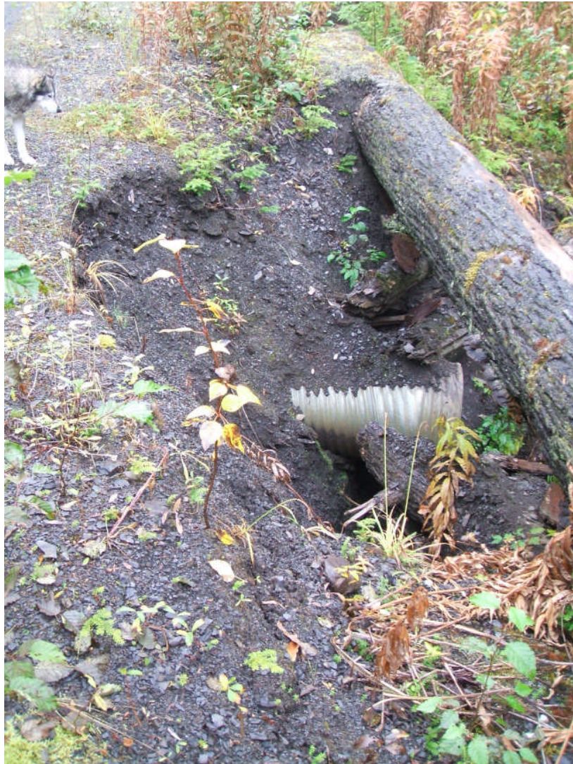
Photo 21: Site 332 – Mass wasting at culvert outlet.
