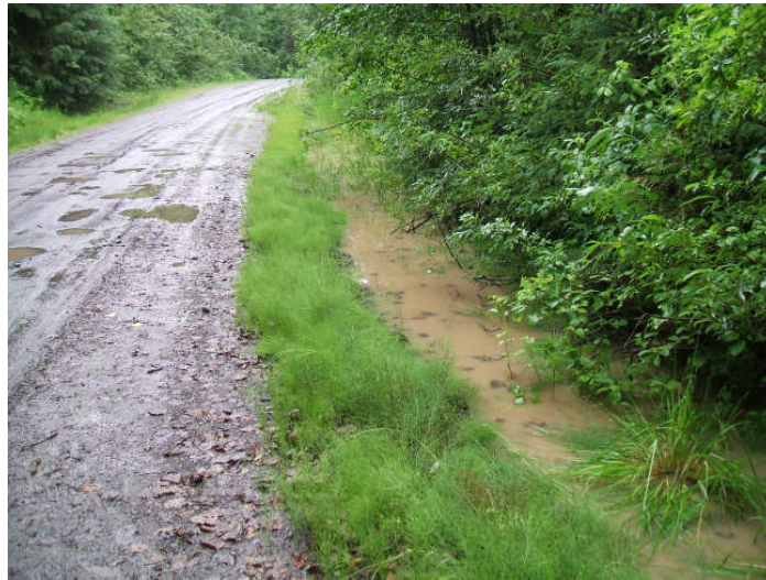
Photo 25: Site 98 – Muddy right-road surface and upper ditch.
