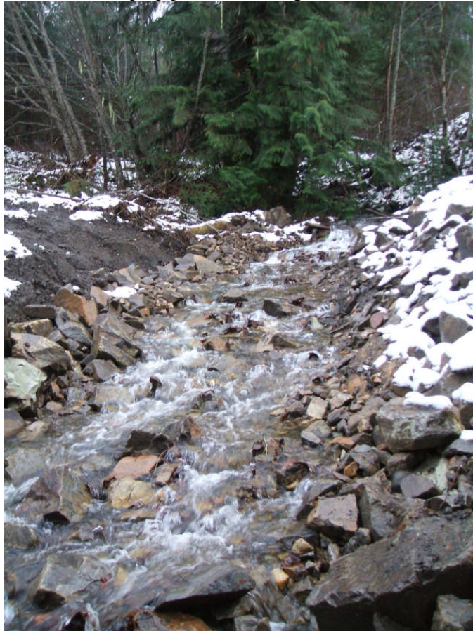
Photo 45: Final riprap placement along new channel at Site 61.
