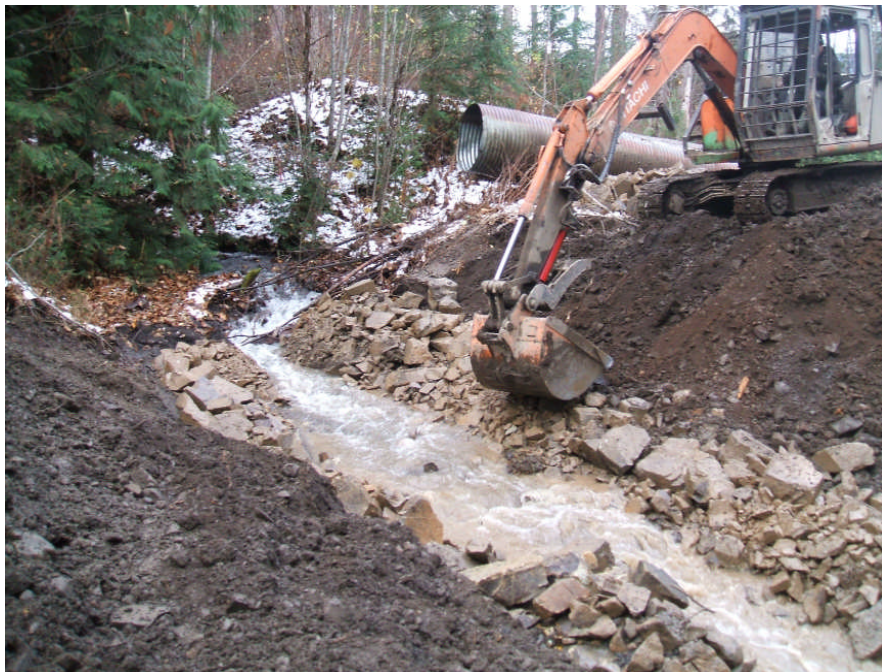
Photo 44: Riprap placement along new channel at Site 61.
