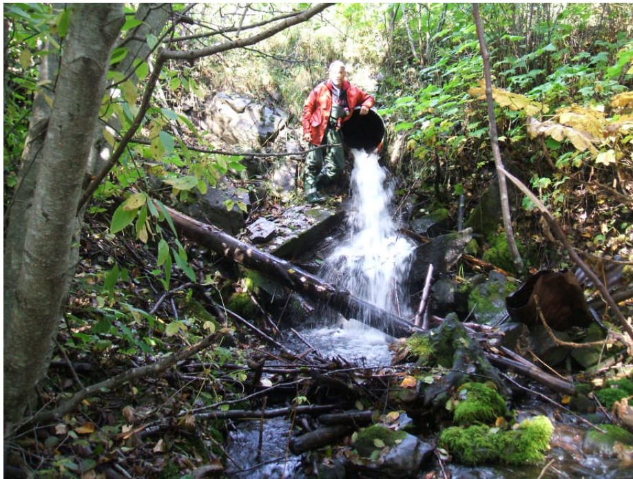
Photo 33: Suspended culvert at Site 47 located along the Mitten Main FSR.
