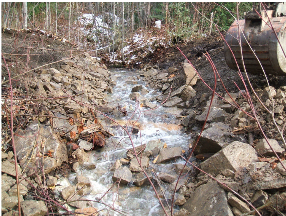
Photo 28: Removing culvert fill material at Site 14.
