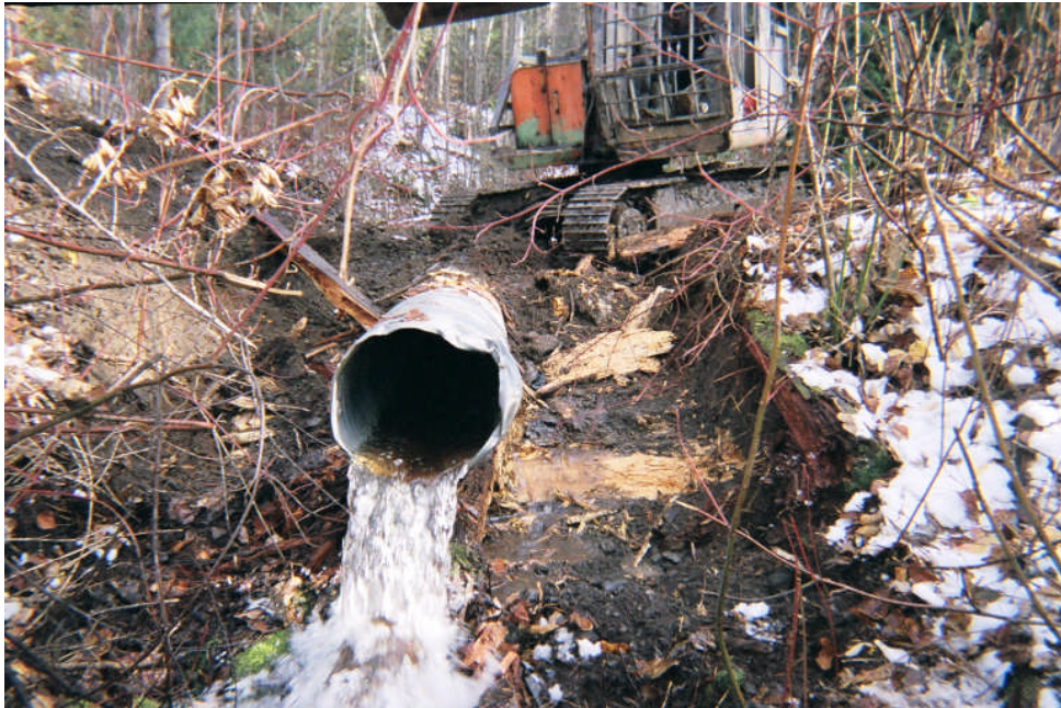
Photo 28: Removing culvert fill material at Site 14.
