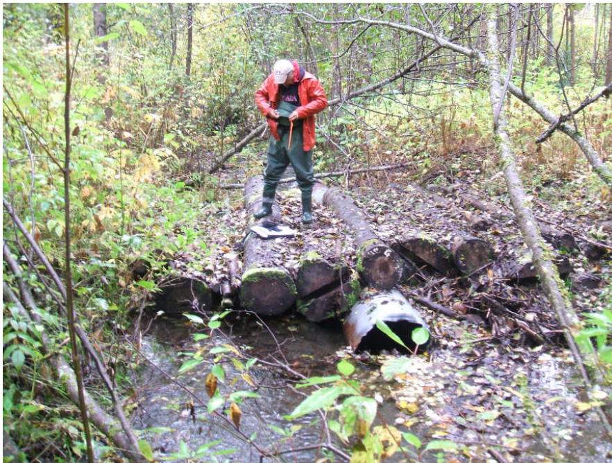
Photo 32: Log fjord and culvert inlet before deactivation.
