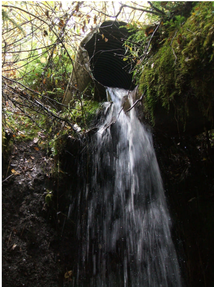
Photo 24: Site 61 – Mass wasting at culvert outlet.
