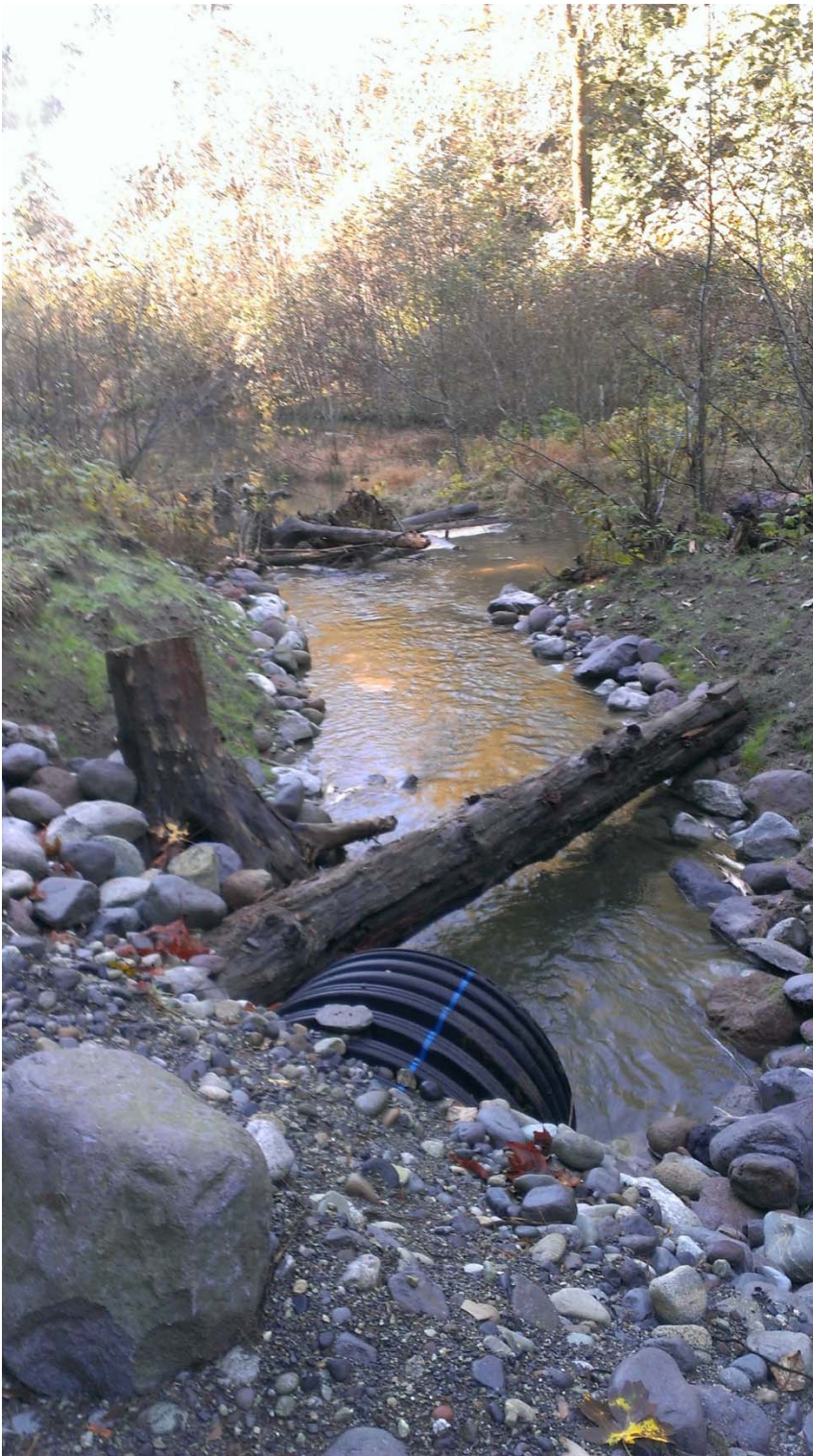
Facing downstream towards the south from same location as photo above. Note LWD placement and large river rock boulders along slopes
