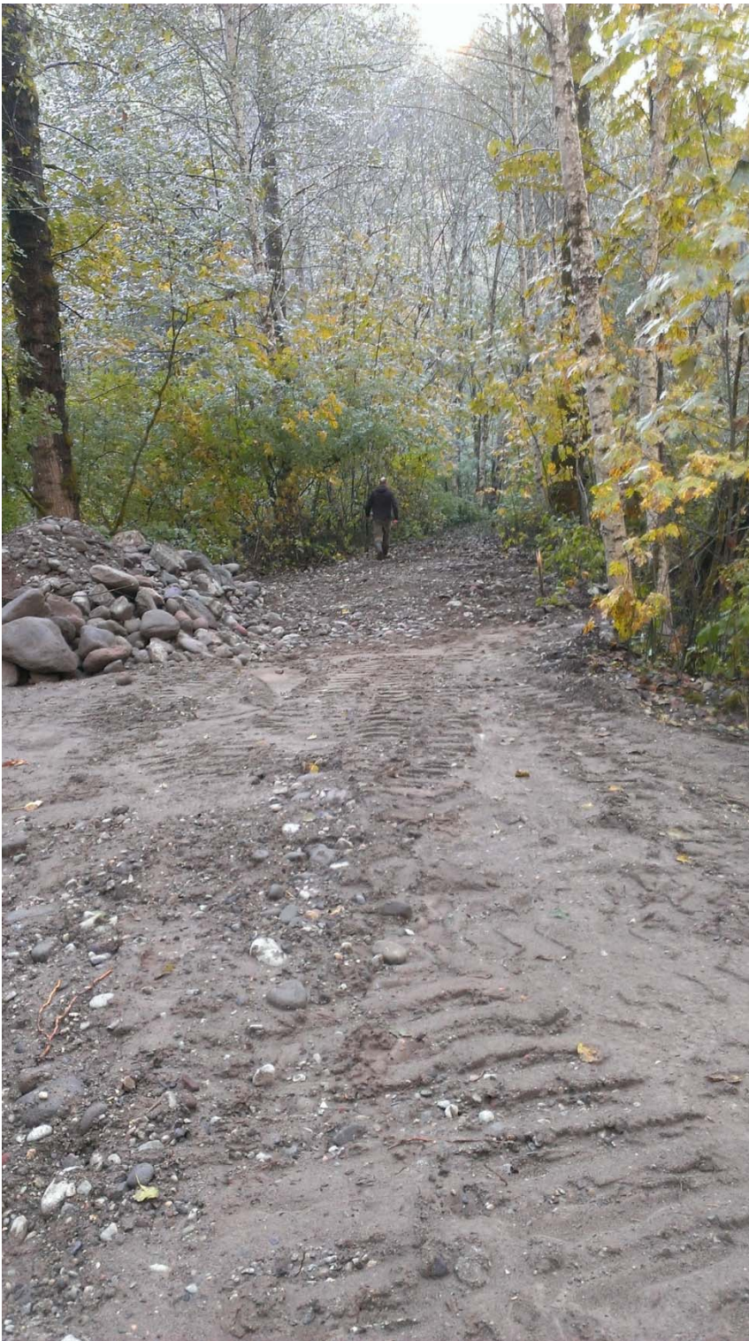
Walking along the dike towards the southern end of the project
