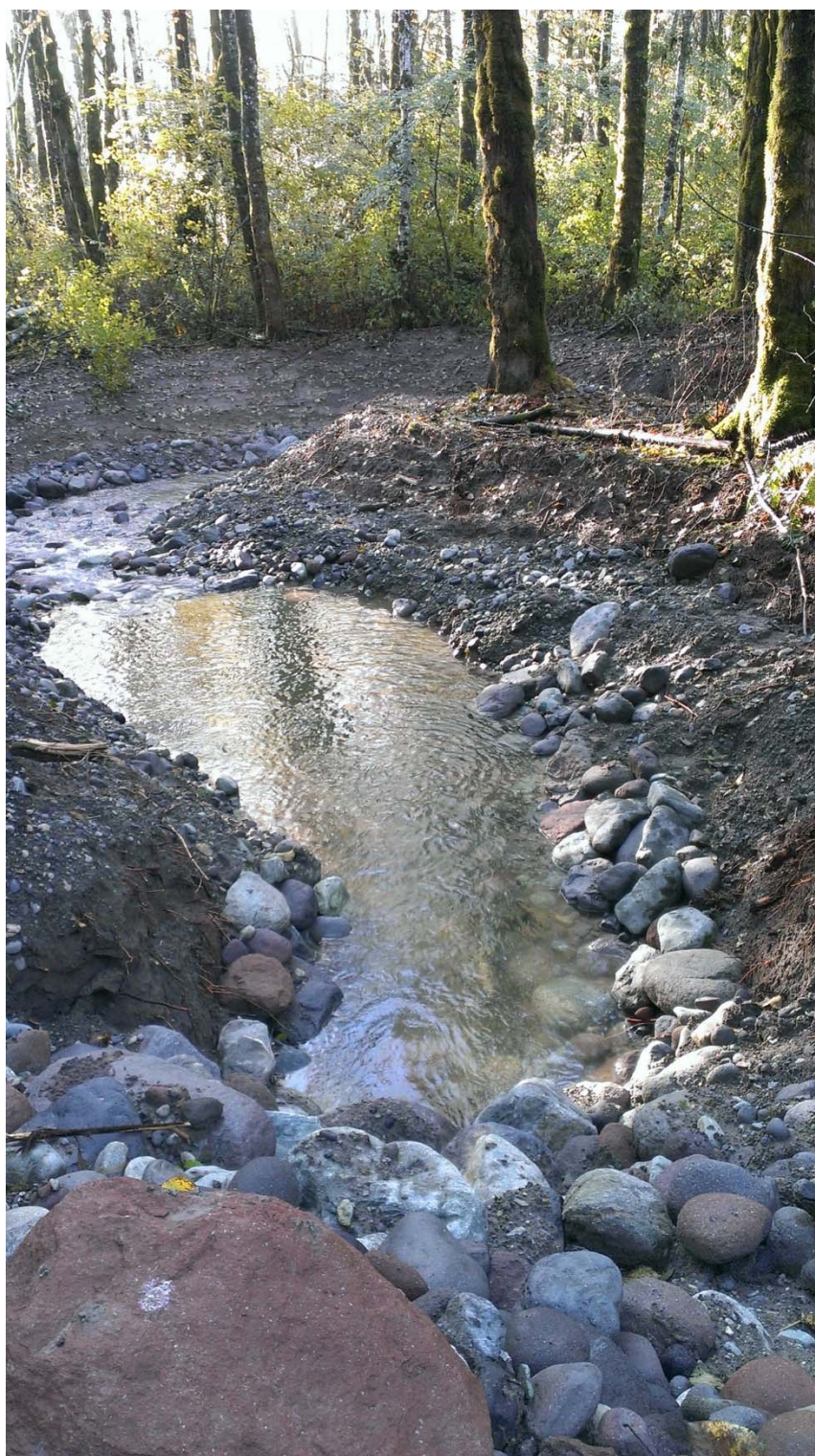
Facing downstream from same location as above photo; note large river rock placement on banks
