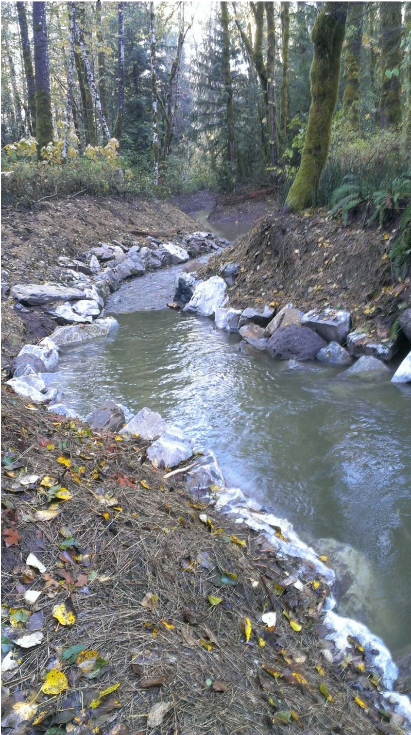
Facing downstream along newly constructed channel – note armoured embankments
