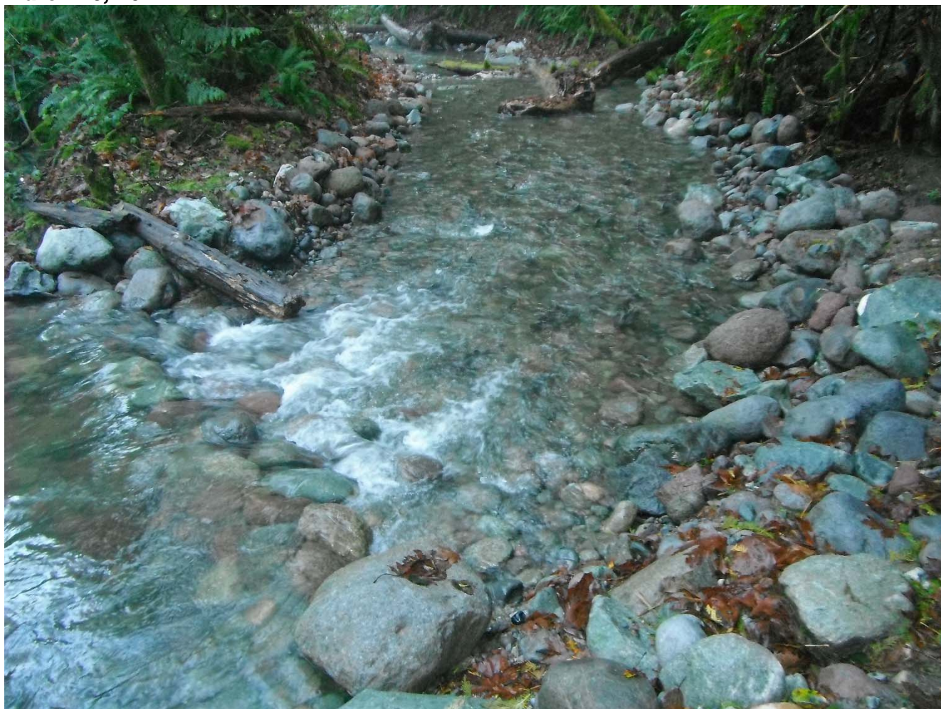
Facing downstream along newly constructed and newly graveled Coho Channel
