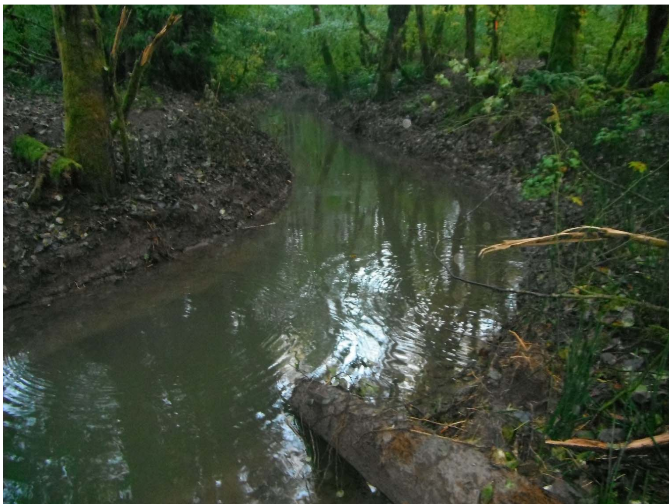
New channel (primary rearing habitat and overwintering for Coho fry) parallel to Moody's Channel on north side of Flood Dyke
