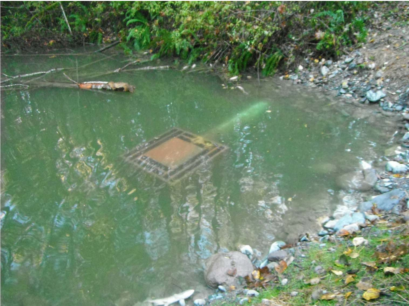
Duck Pond Intake (installed March 24, 2014)
