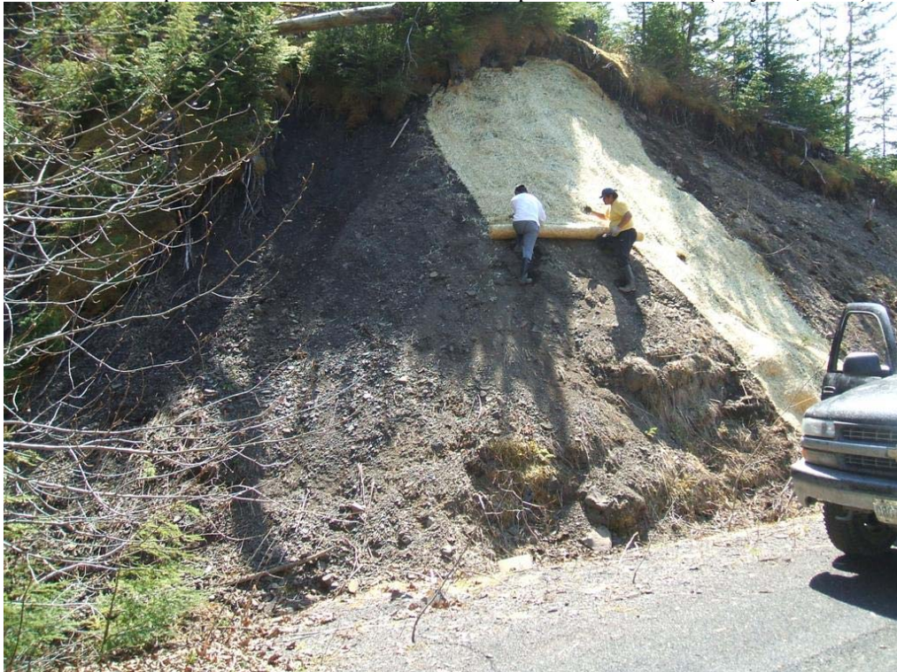
Photo 27: GFA crew applying ECBs at Site 42 (May 26, 2008).
