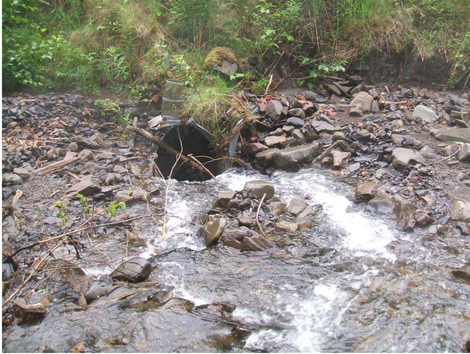
Photo 2: Partially blocked left culvert intake and completely blocked right culvert intake at Site 91 prior to deactivation.
