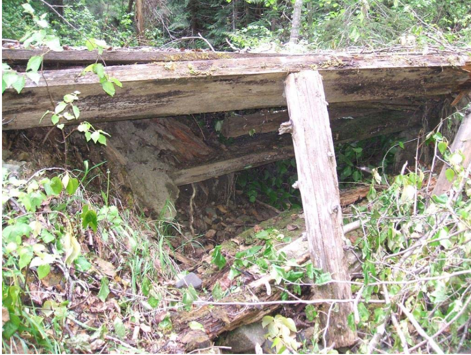
Photo 70: Collapsing bridge deck at Site 347 (11 Mile Road Branch).
