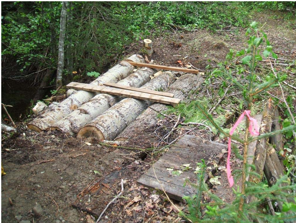
Photo 71: Recently constructed ATV crossing at Site 347.
