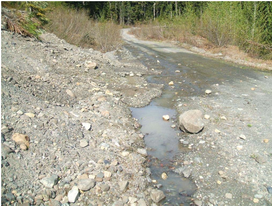
Photo 35: Ditch covered with cutbank sediment and water flowing over road surface at Site 186 (May 27, 2008).
