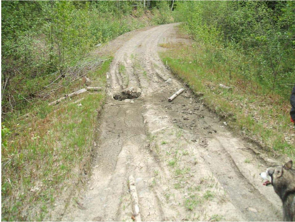
Photo 55: Wood box culvert collapsing into stream at Site 21.
