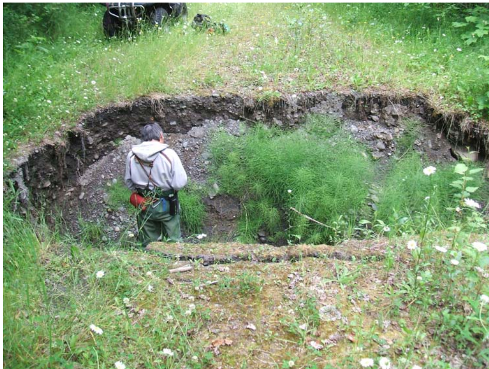
Photo 86: Large hole from collapsed wood-box culvert along Wagon Creek Road Km 3.4.
