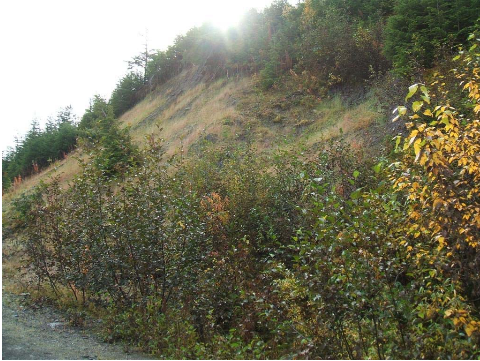
Photo 34: Partially vegetated right road cutbank following treatment (looking away from stream, October 1, 2008).
