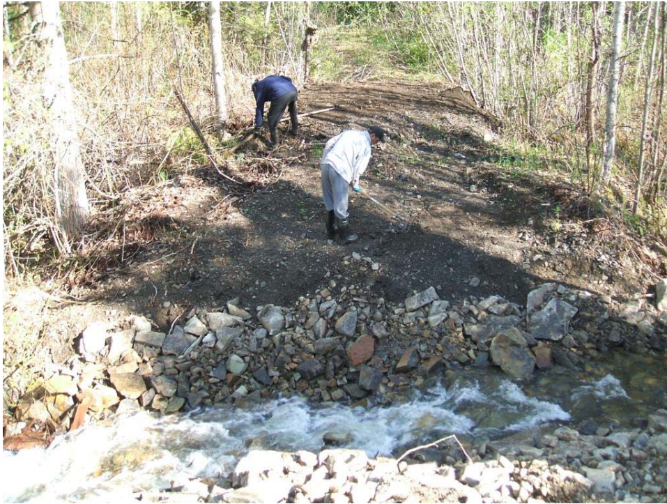
Photo 18: Preparation of exposed right bank and piled road fill prior to treatment at Site 14 (May 22, 2008).
