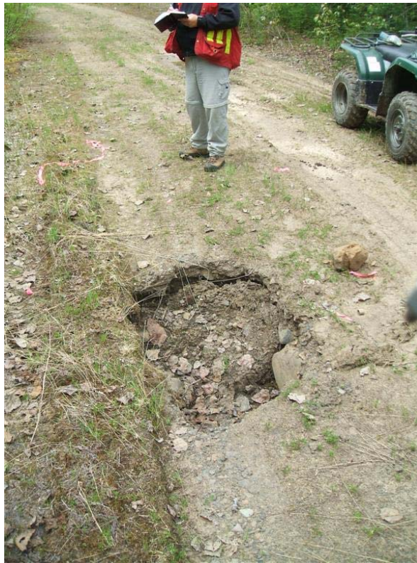
Photo 58: Collapsing wood box culvert at Site 277.
