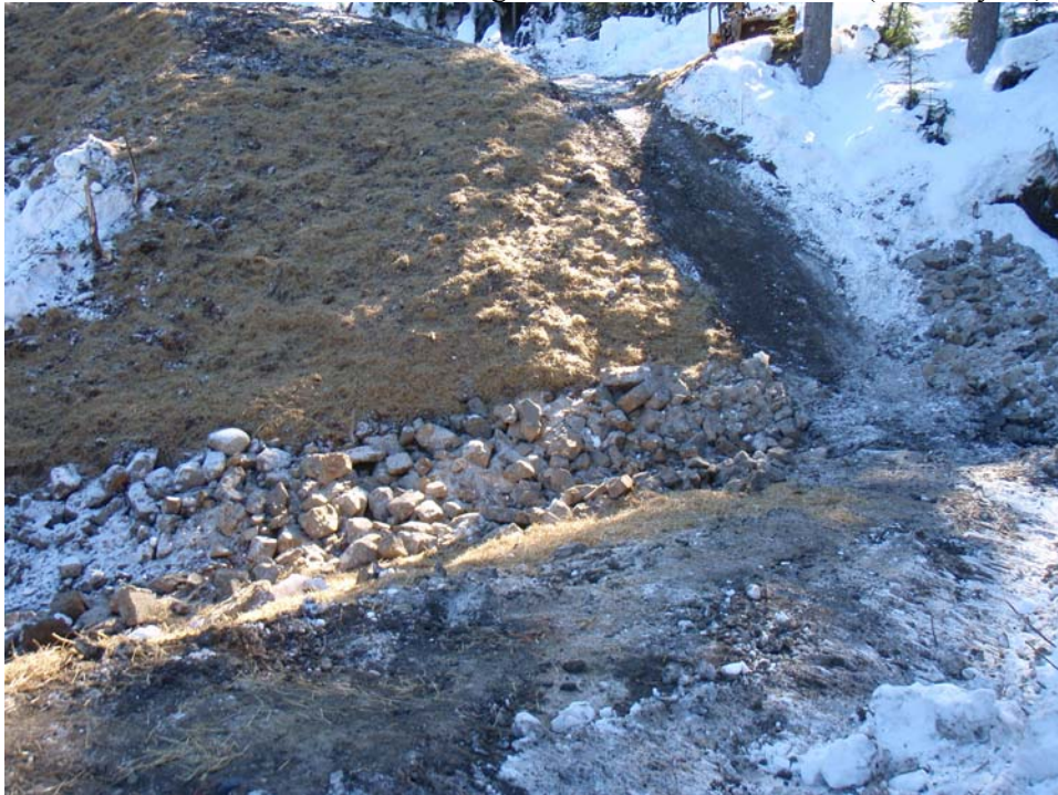
Photo 9: Grass seed and straw mulch applied to the stream banks following the deactivation of Site 91 (February 25, 2009).
