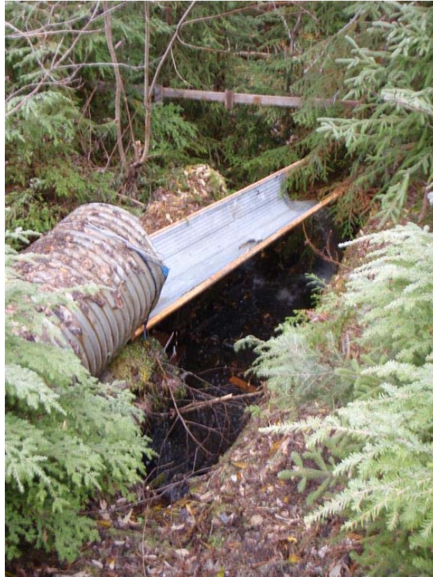
Photo 53: Diversion trough constructed to bypass water away from Site 60.
