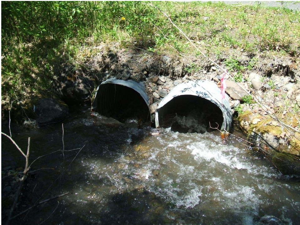
Photo 60: Partially plugged culvert inlets at Site 3 (Chernobel Creek).
