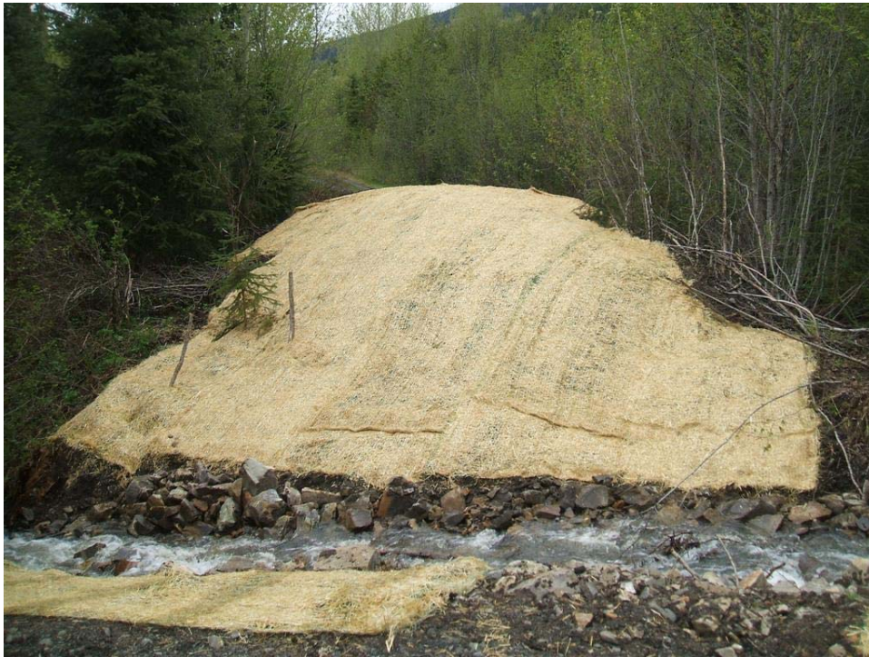
Photo 12: Right bank seeded and covered with ECBs at Site 61 (May 22, 2008).
