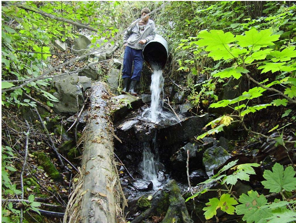
Photo 74: Site 47 looking upstream at suspended outlet.
