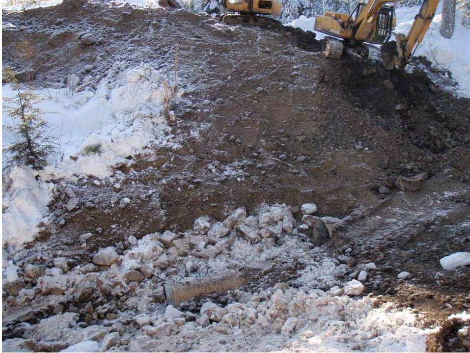
Photo 6: Removal of culverts and armoring of stream banks at Site 91 (February 11, 2008).
