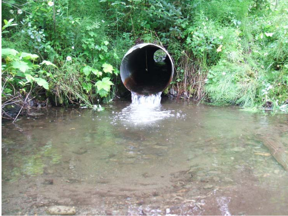
Photo 81: Suspended culvert outlet at Site 59, Wagon Creek Road.
