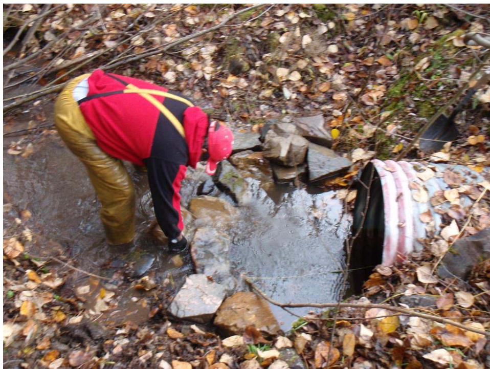
Photo 68: Hand placement of rock levee at Site 61.
