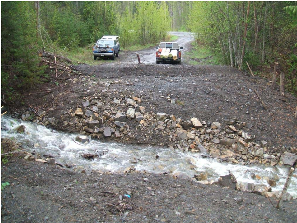
Photo 14: Exposed left bank following the 2007 deactivation of Site 61 (May 22, 2008).
