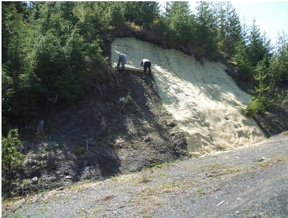
Photo 24: GFA crew applying ECBs at Site 35 (May 26, 2008).
