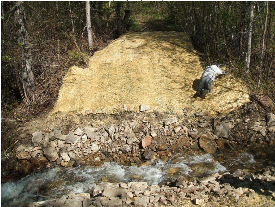
Photo 19: Right bank seeded and covered with ECBs at Site 14 (May 22, 2008).
