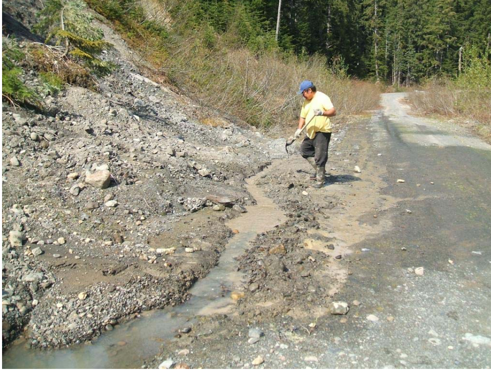
Photo 36: GFA digging a temporary ditch at Site 186 prior to direct water into a series of small retention ponds (May 27, 2008).
