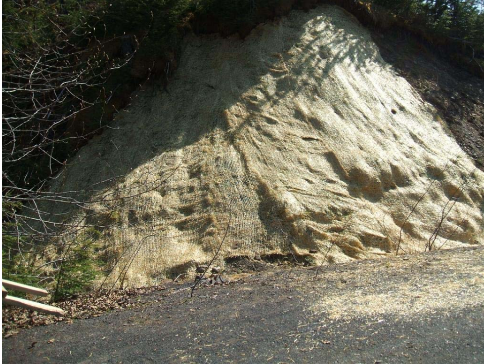
Photo 28: Left bank seeded and covered with ECBs at Site 42 (May 26, 2008).
