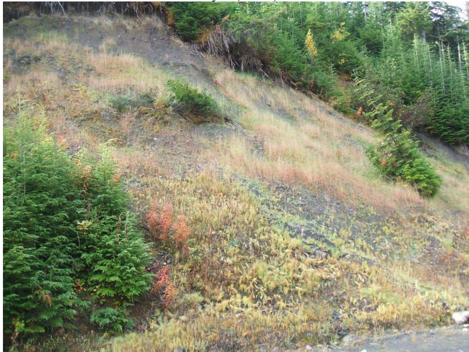
Photo 33: Partially vegetated right road cutbank following treatment (looking towards stream, October 1, 2008).
