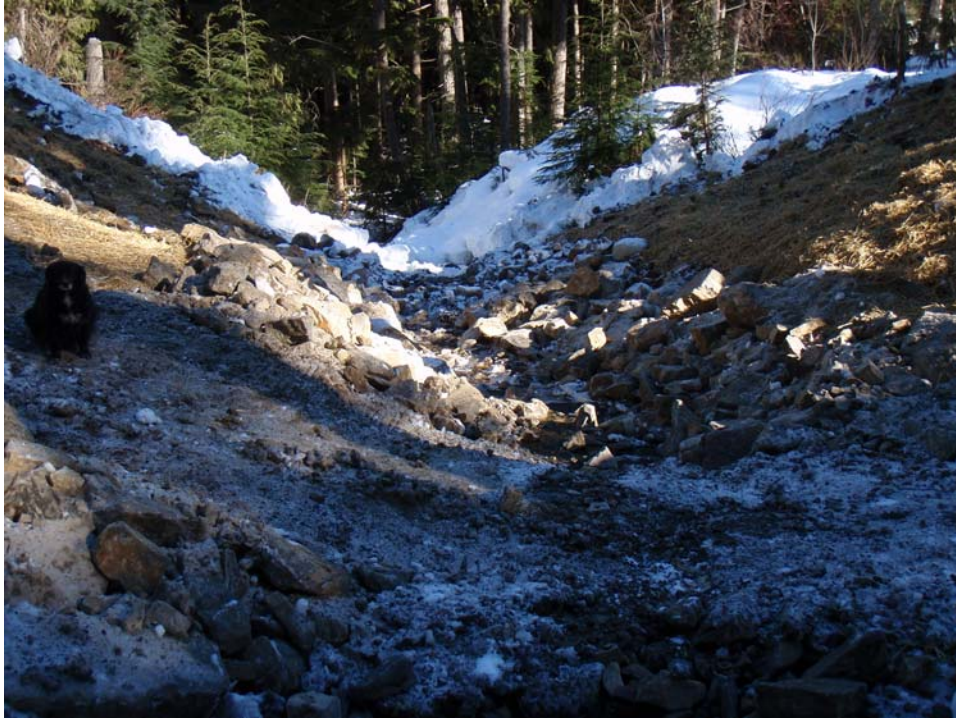
Photo 8: Armored stream channel following the deactivation of Site 91 (February 25, 2009).
