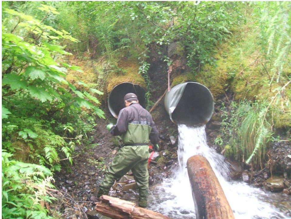
Photo 1: Suspended culvert outlets at Site 91 prior to deactivation.
