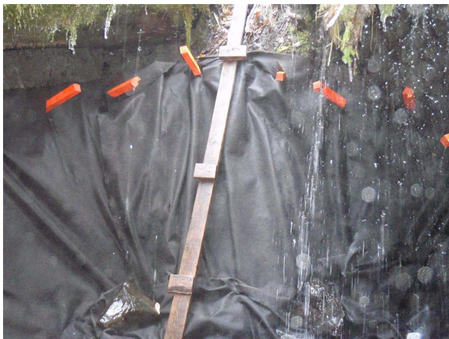
Photo 54: Eroding stream bank covered with Geotextile at Site 60.
