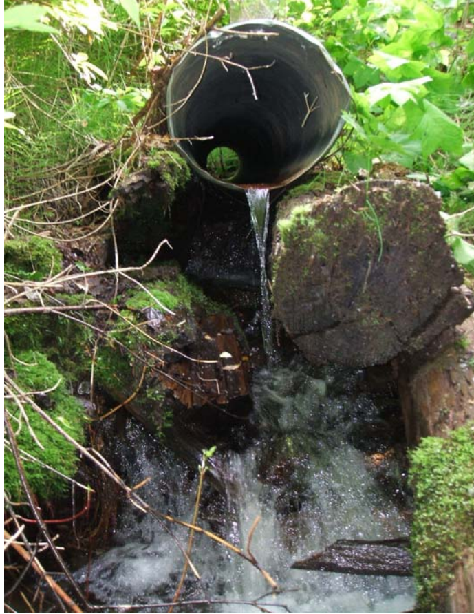
Photo 16: Suspended culvert at Site 14 prior to deactivation (October 2007).
