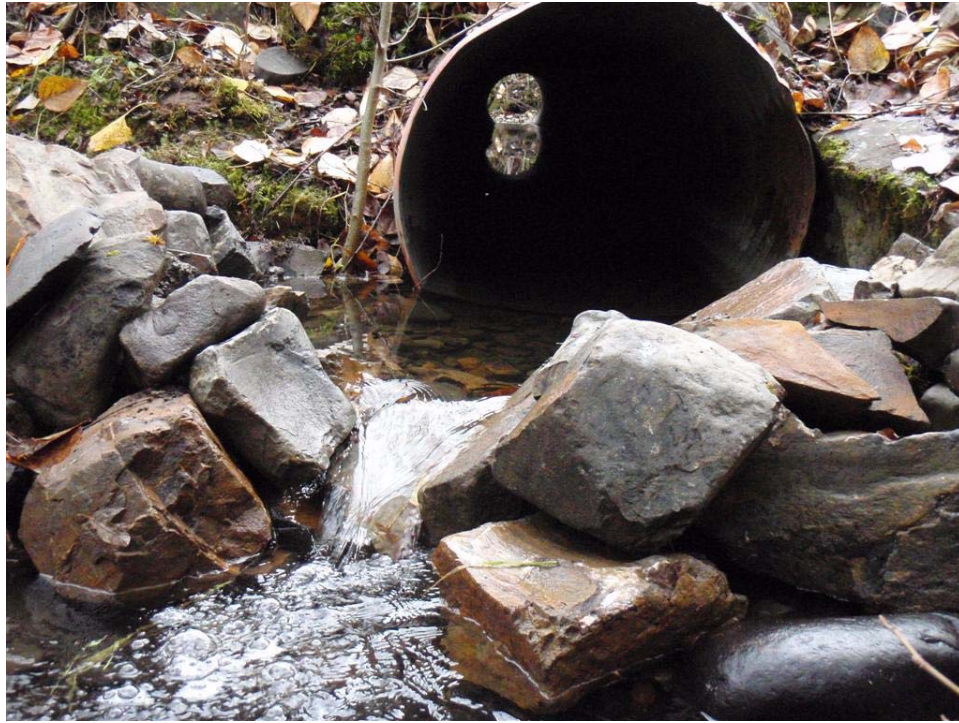
Photo 69: Rock levee and backwatered culvert following treatment of Site 61.
