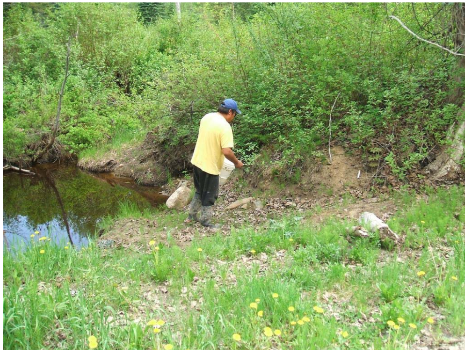
Photo 41: GFA crew applying grass seed and fertilizer to Site 270 (May 27, 2008).
