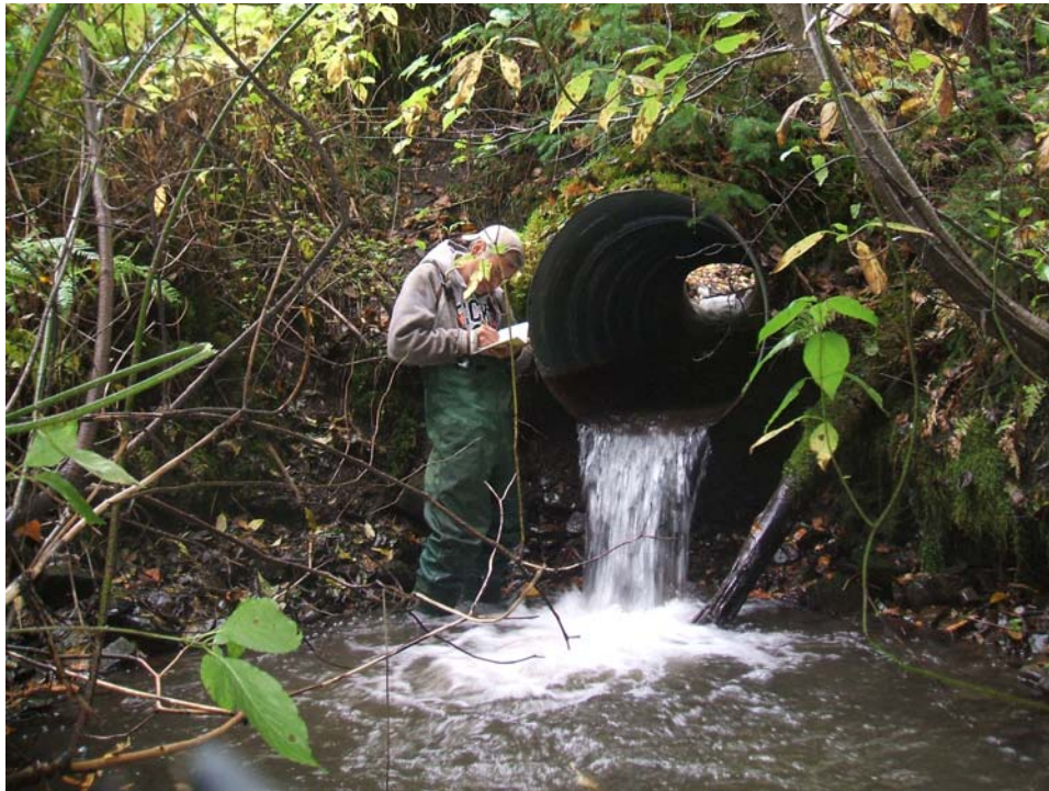
Photo 10: Suspended culvert outlet at Site 61 prior to deactivation (2006).
