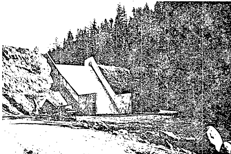
Figure No. 10 - Storage dam under construction on Vernon Creek, September 1970.
