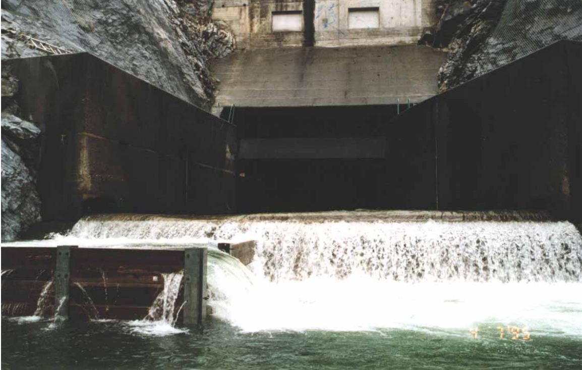
Plate 9. Fish attracting flow from the flip bucket showing function of the fish weir.
