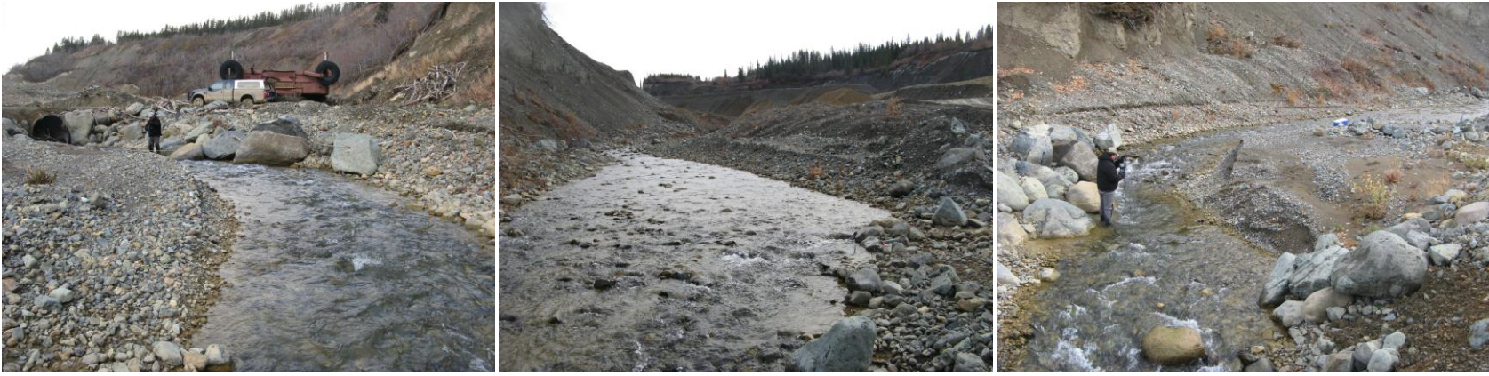
FIGURE 35 Downstream (DS) Spruce Creek sample location looking downstream (note the culvert), a view upstream from the same location, and a view upstream from the culvert. The Pictures were taken while gravel washing took place and no surface discharge was observed.
