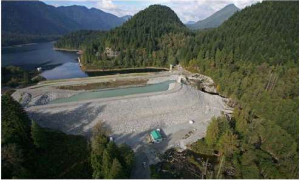
Figure 2 Picture of Coquitlam Dam (Stuart 2010).
