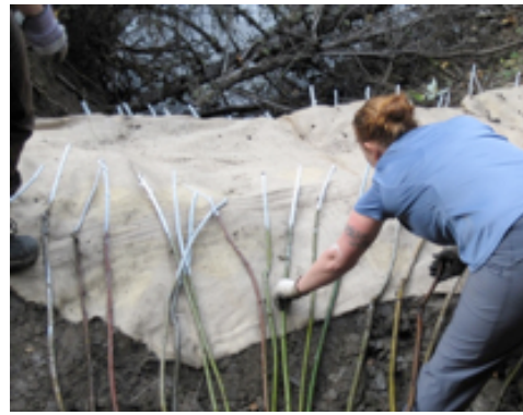
Figure 16- Live cuttings were planted between layers of coir erosion control cloth
