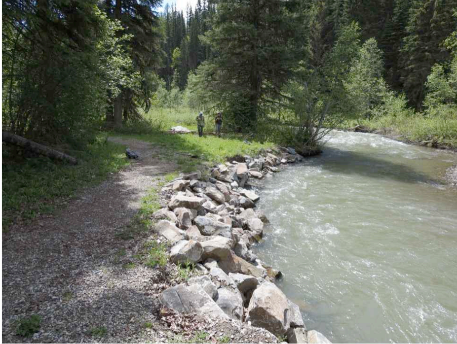
Figure 3 – Photo of Site 1 Rip Rap restoration site, July 2014
