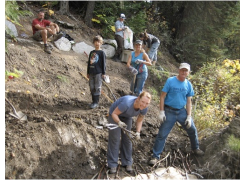
Figure 15- Field crew installing live cuttings
