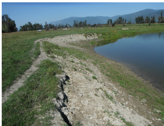
Photo 8. Exposed soils at cattle access point September 11, 2013.
