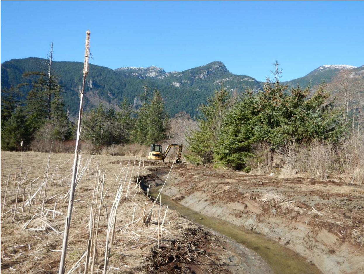
Photo 14. March 7, 2015 – Constructing new tidal channel – facing west
