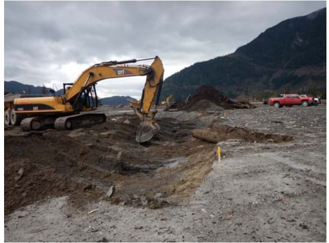
Photos 6 & 7: March 2015. Site excavation – right photo including central tidal channel construction
