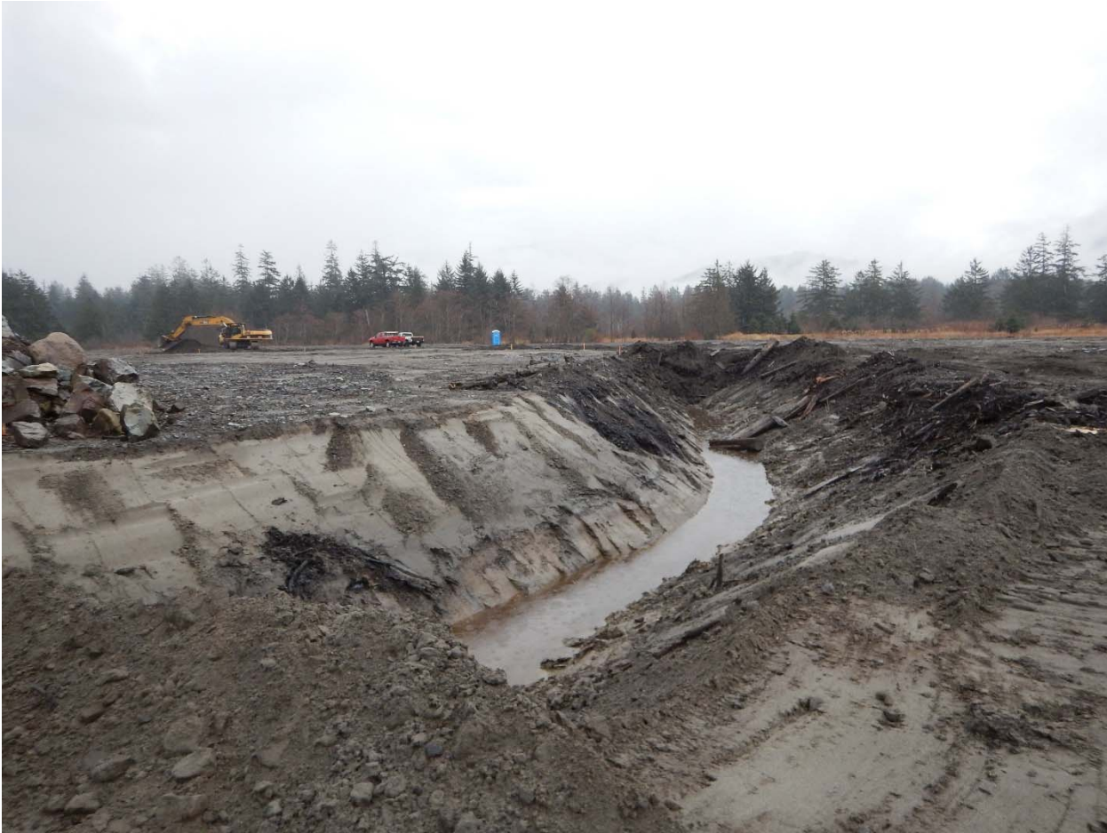
Photo 15. April 11, 2015 – Facing east. Constructing large tidal channel at south end
