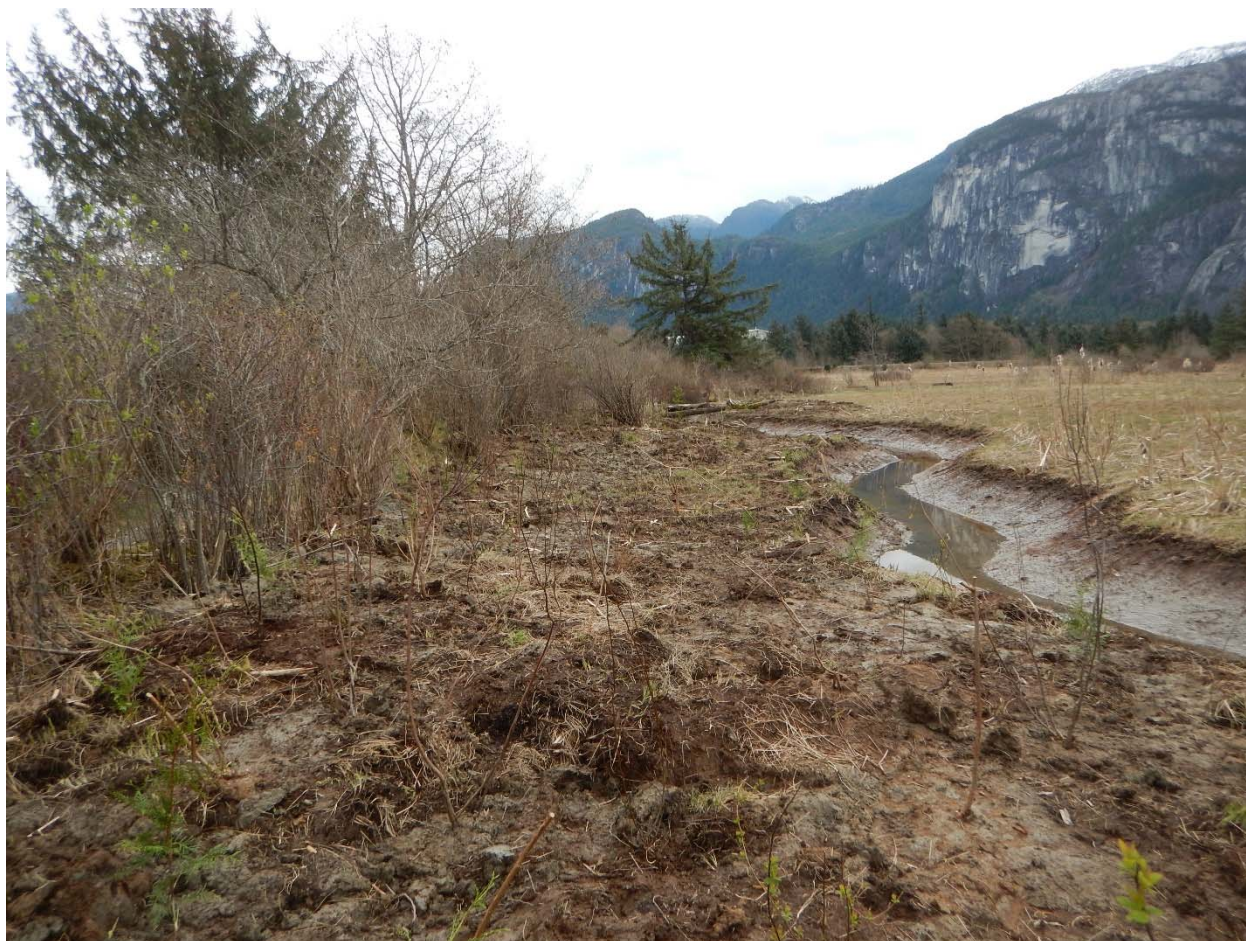
Photo 19. May 22, 2015 – top end of completed southern tidal channel – note riparian vegetation planted by volunteer support
