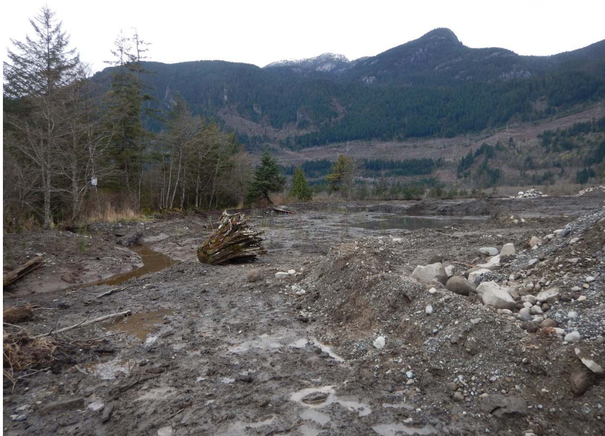
Photo 18. April 22, 2015 – Completed tidal channel at south end of site (lower section)
