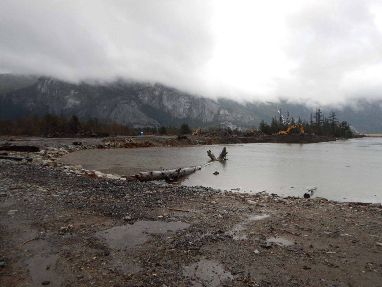
Photo 16. April 14, 2015 – facing east towards construction (note in-filling of log-dump pond)
