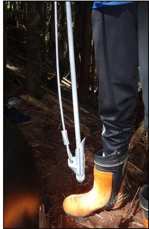
Figure 4. Cable anchor on pounding rod before installation.
