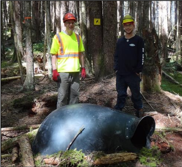
Figure 7. Rob Martin (BCTS) and Cory Cliffe after installing den pod CR002.
