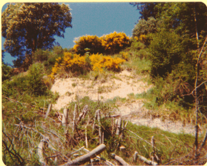
3619 Farhill Road, Metchosin, B.C. West of A. Webster's Property May 1977 Gravel Pit Development Complaint
