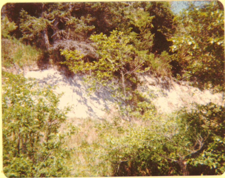
3619 Farhill Road, Metchosin, B.C. Further east on Beach trail from A. Webster's Property May 1977 Gravel Pit Development Complaint
