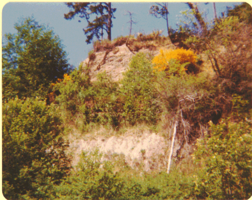
3619 Farhill Road, Metchosin, B.C. East of A. Webster's Property May 1977 Gravel Pit Development Complaint
