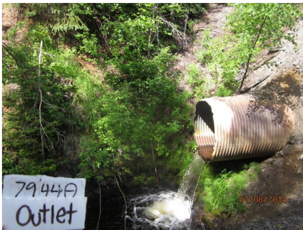
Photo 29, Site 7944A – 1.2m perched culvert.
