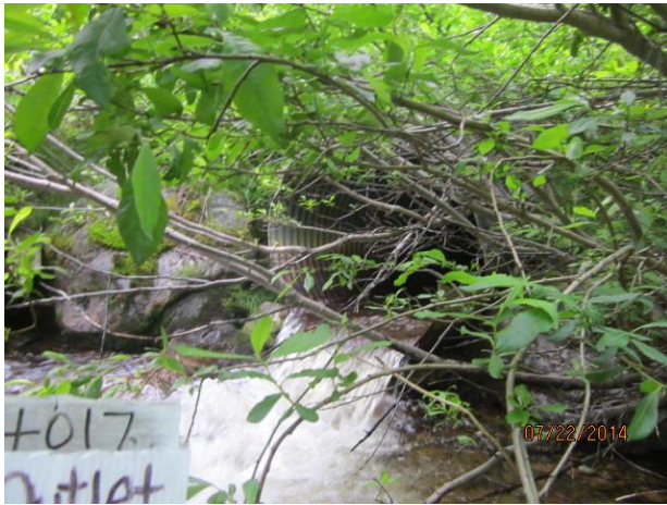
Photo 25, Site 4017 – Outlet perched 0.6m.
