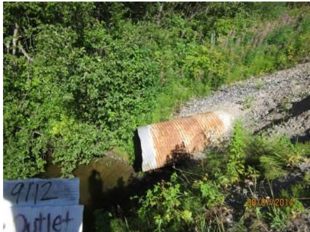
Photo 17, Site 9112 – 0.61m perched outlet.
