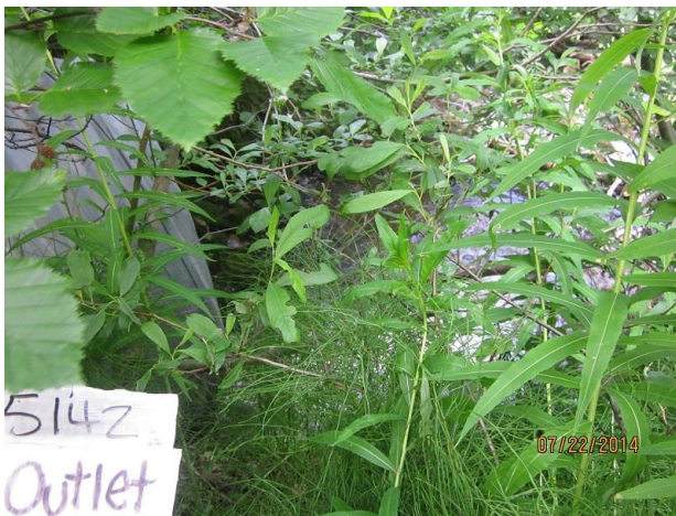
Photo 27, Site 5142 – Outlet perched 0.6m.
