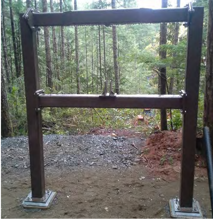
Photo 13. Erected South Tower structure, March 18, 2016.
