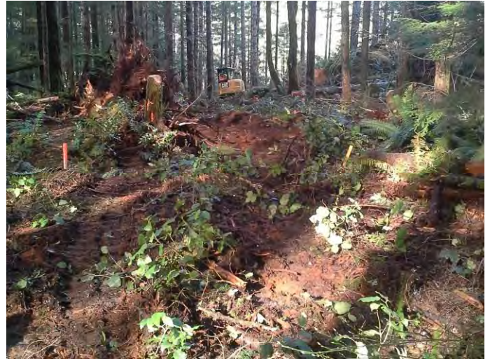
Photo 6. Clearing trail right of way and South Tower location, February 24, 2016.
