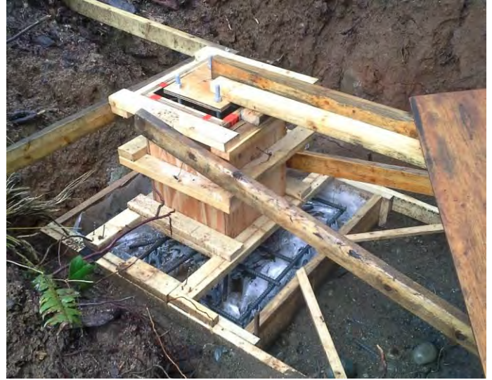
Photo 10. Forms for South Tower footing, March 3, 2016.
