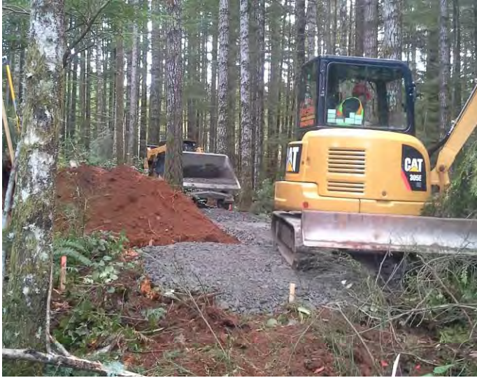
Photo 9. Excavation for South Tower footings and winch pad, February 25, 2016.
