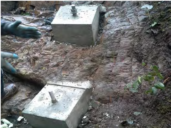
Photo 11. North side anchors, drilled and cast March 9, 2016.
