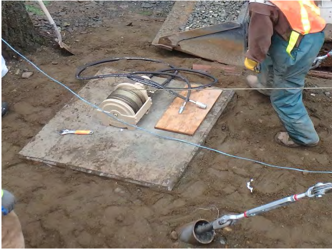
Photo 17. Hydraulic winch installed on concrete winch pad, March 24, 2016.
