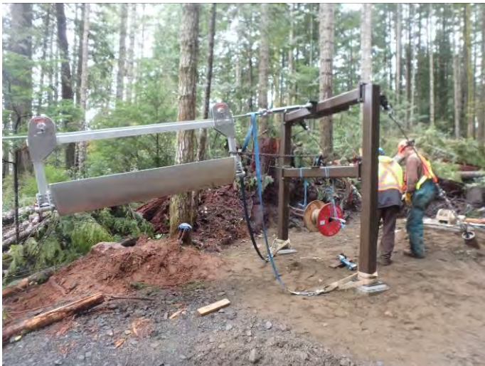
Photo 15. Fully installed south tower and gravel trolley ready for testing, March 24, 2016.
