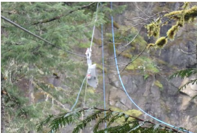
Photo 19. Gravel trolley bucket mid release, first test March 24, 2016.
