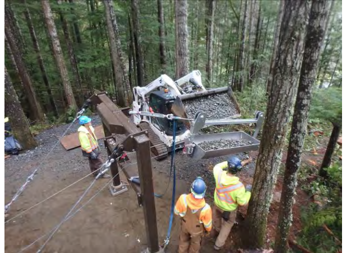
Photo 18. Loading the trolley bucket with washed spawning gravel for test release, March 24, 2016.
