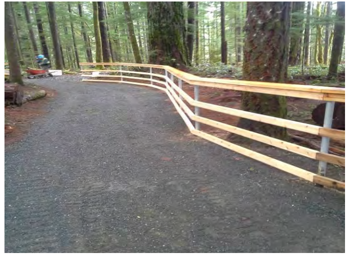
Photo 12. Newly constructed cedar fencing along Millennium Trail, March 10, 2016.
