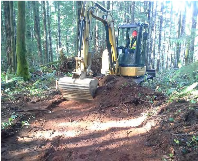
Photo 7. Removing overburden for access trail February 24, 2016.
