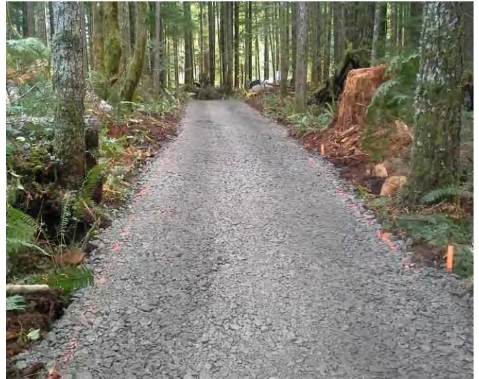
Photo 8. Newly constructed access trail to South Tower location of compacted '3 inch minus' fractured rock, February 25, 2016.
