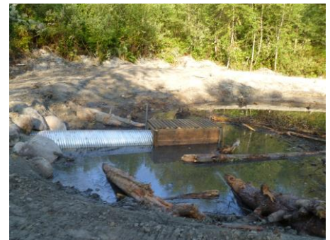
Archery Pond and Off-channel Habitat Project Beaver Resistance Culverts
