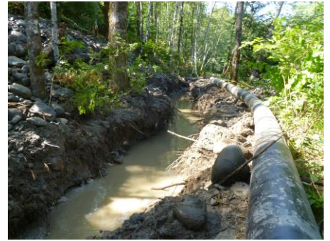
Archery Pond and Off-channel Habitat Project New 108m Waterline
