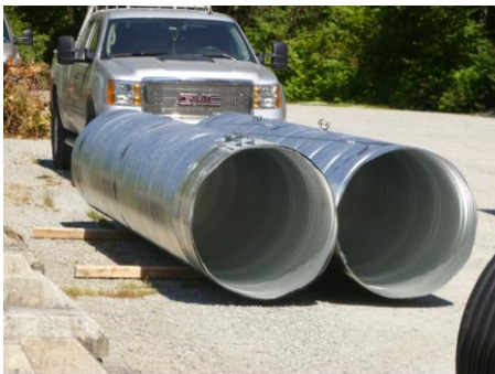
Archery Pond and Off-channel Habitat Project Beaver Resistance Culverts
