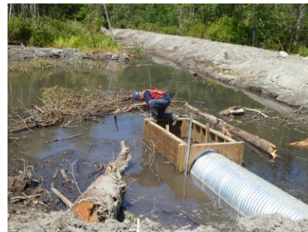
Archery Pond and Off-channel Habitat Project Beaver Resistance Culverts
