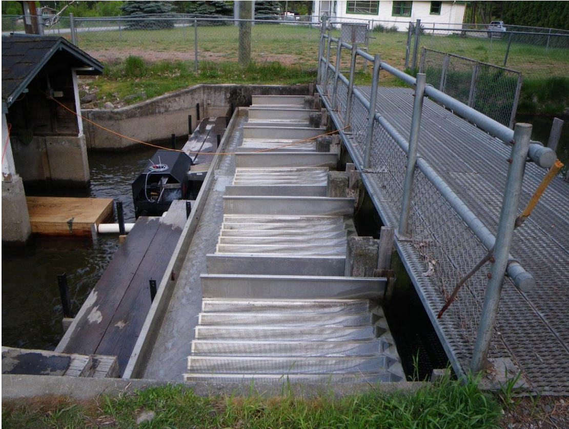
Figure 3. Weir at the Gates Creek spawning channel. Fish are funnelled through the black sampler structure in the middle of the trough to the wood box visible on the left.
