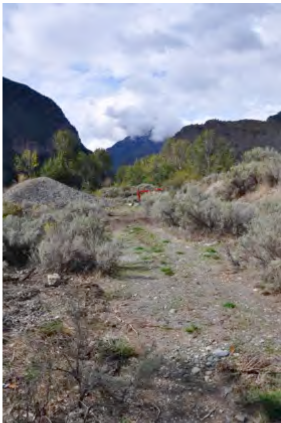
Figure 52 Excavator preparing old road and gravel berm site Lower Spawning Channel
