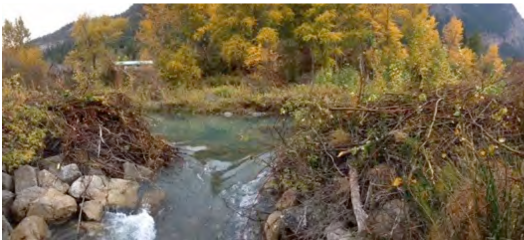
Figure 22 Beaver dam removed 19 Oct 2015
