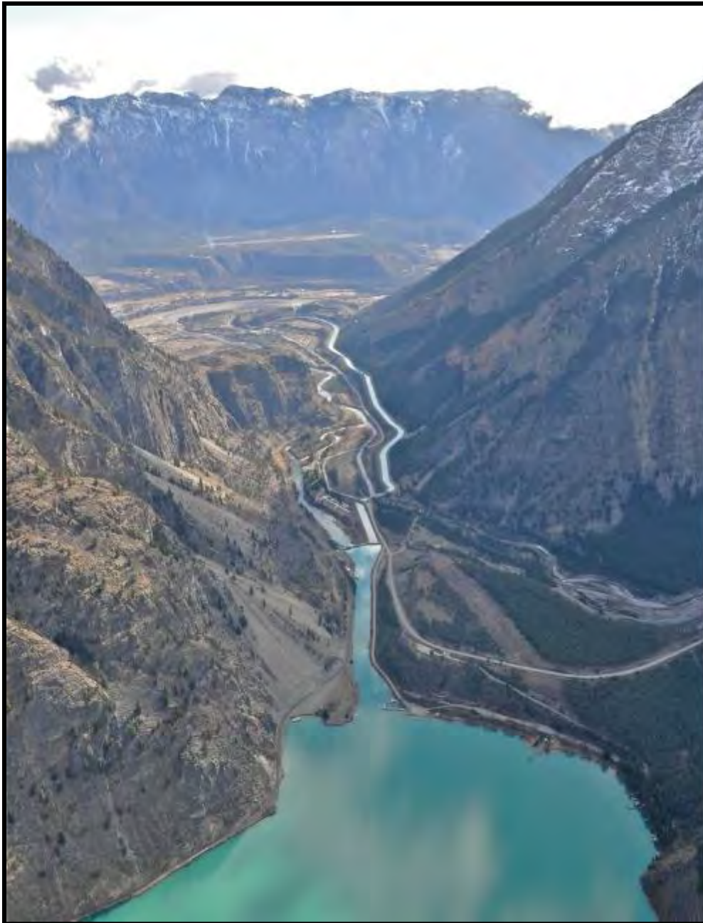
Figure 2 Aerial photograph showing the narrow valley and some of the impacts 29 Mar 2011
