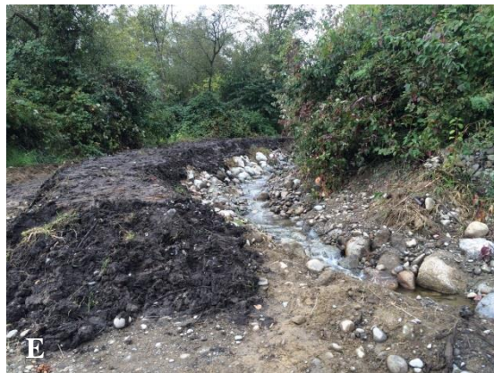
A. Excavator digs out sediment from fishway. B. Fishway before restoration-completely de-watered, C. Fishway after restoration. D. Thompson creek channel and riparian damaged and dried out. E. During works, spoil was used to create a berm and riparian habitat along Thompson Creek. F. Replanted berm with signage informing people to care for this habitat.
