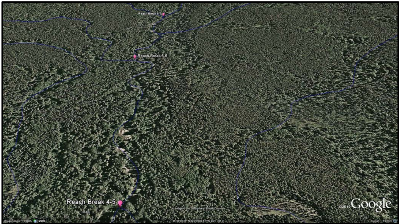
Figure 7. Google Earth image looking upstream along Reaches #5 and 6 of Sandpoint Creek.
