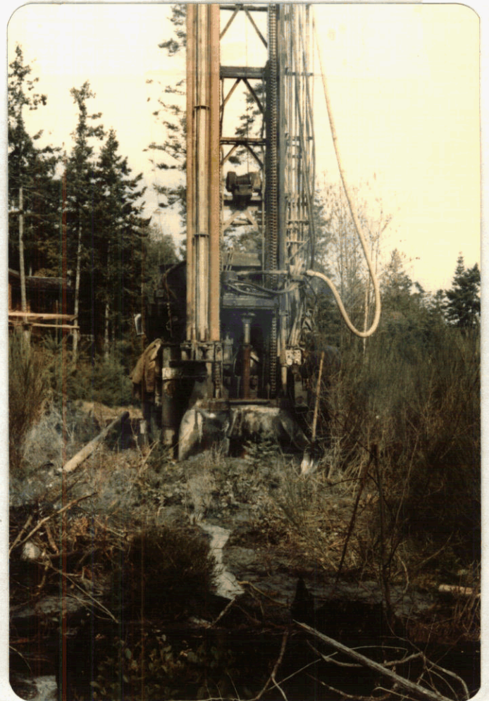
3. Observation Well WR 258-60 Galiano Island (south) Drilling in progress
