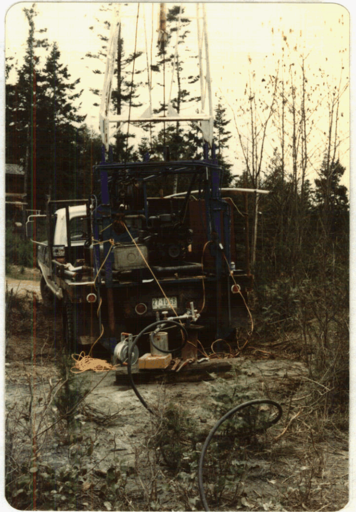
5. Observation Well WR 258-60 Galiano Island (south) Pumpint test equipment set-up.
