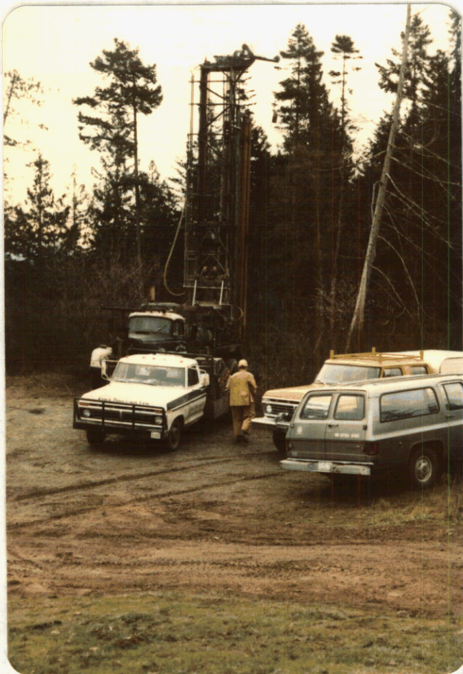
2. Observation Well WR 258-60 Galiano Island (south) Ken's Drilling setting up
