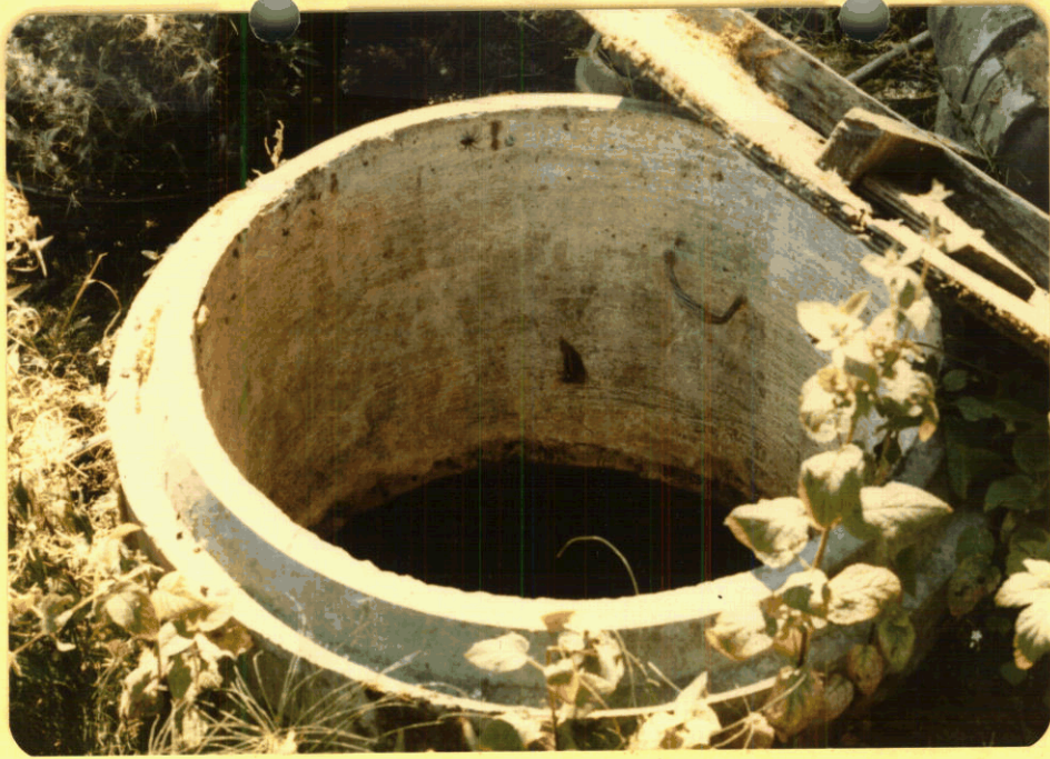
Concrete Cribbing (30") Retaining Spring water 8' west of slump- 40' from Isabella Point Rd
