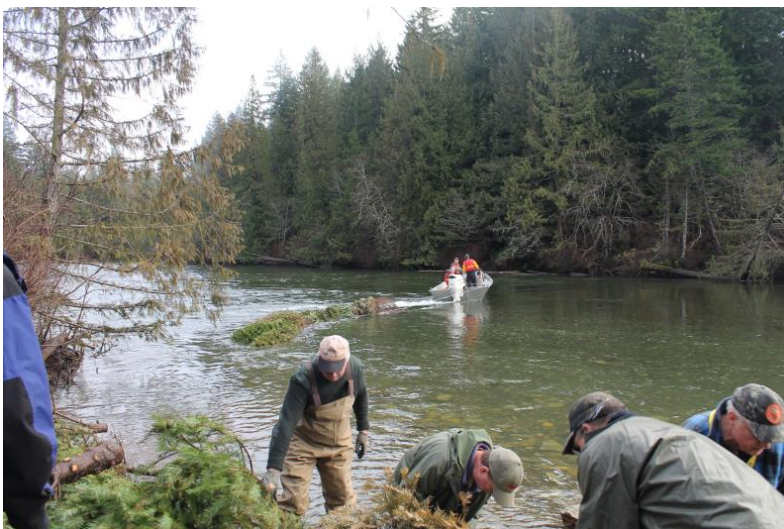
Photo 14. Towing completed SWD bundle to receiving site downstream.
