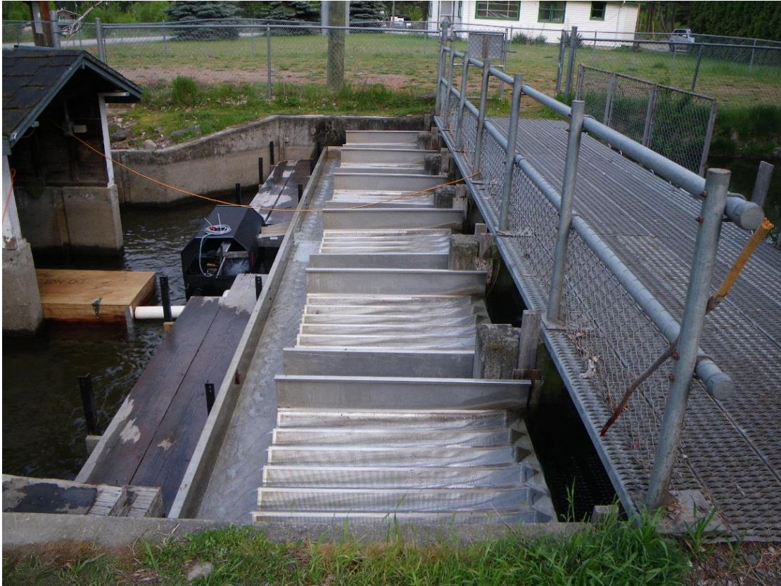
Figure 3. Weir at the Gates Creek spawning channel. Fish are funnelled through the black sampler structure in the middle of the trough to the wood box visible on the left.
