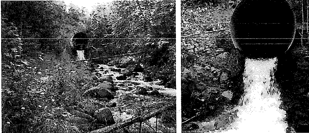
Photo 1 and 2. Looking upstream to the outlet
