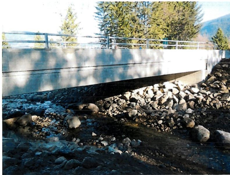
Figure # 2 – New Bridge over Highway 6 – September 2016
