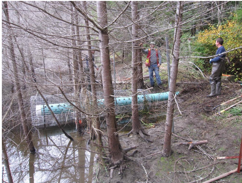
Photo 5. Example of a beaver pond level control pipe for possible future installation at Forbidden side-channel (photo credit M. Sheng).
