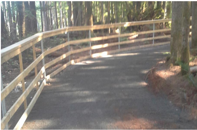
Photo 9. Repaired millenium trail at the end of the project.
