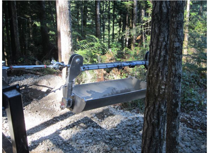
Photo 2. Gravel trolley installed on overhead cable, ready for loading
