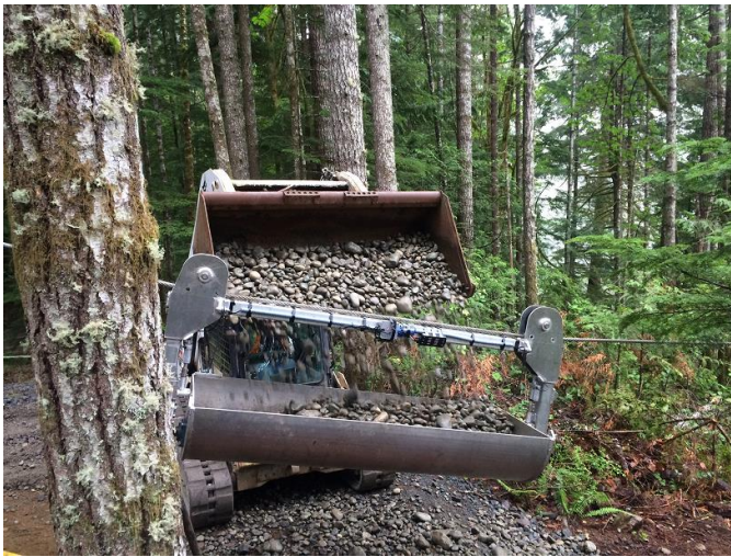
Photo 7. Loading trolley bucket with skidsteer.
