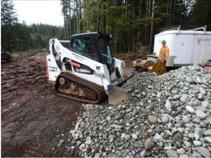
Photo 5. Gravel staging area.
