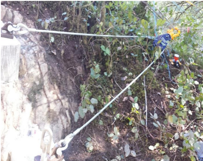
Photo 3. North anchor bridle system.
