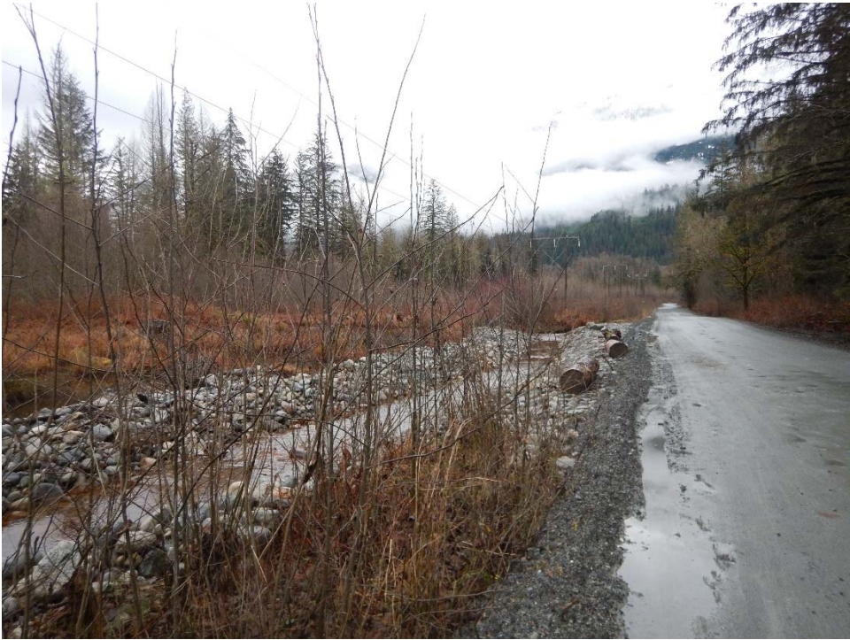
Facing east towards “Culvert 2”
