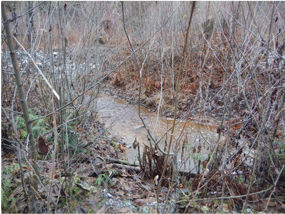
“Culvert 1” – facing north, upstream of road
