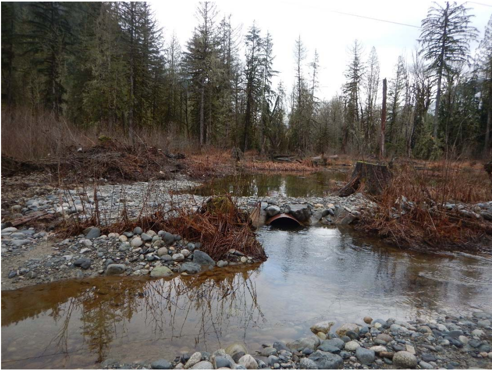
Facing north towards new culvert/berm between "Culvert 3" & "Culvert 4"
