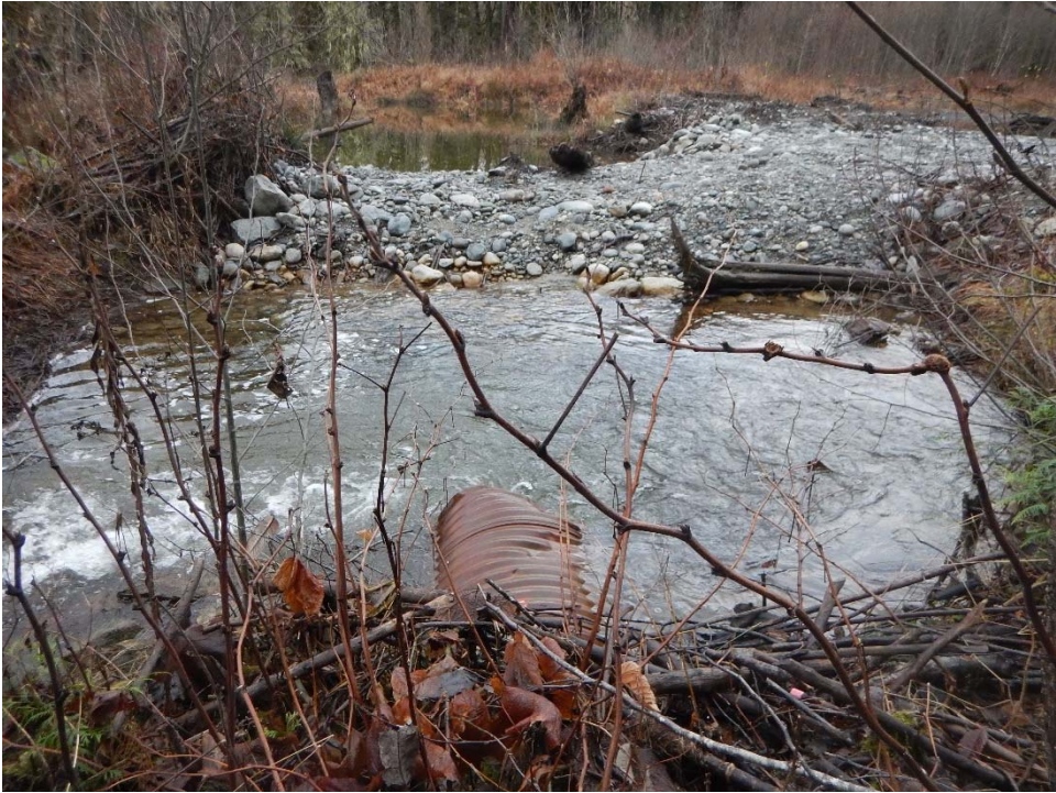
“Culvert 3” – facing north, upstream of road; note gravel berm
