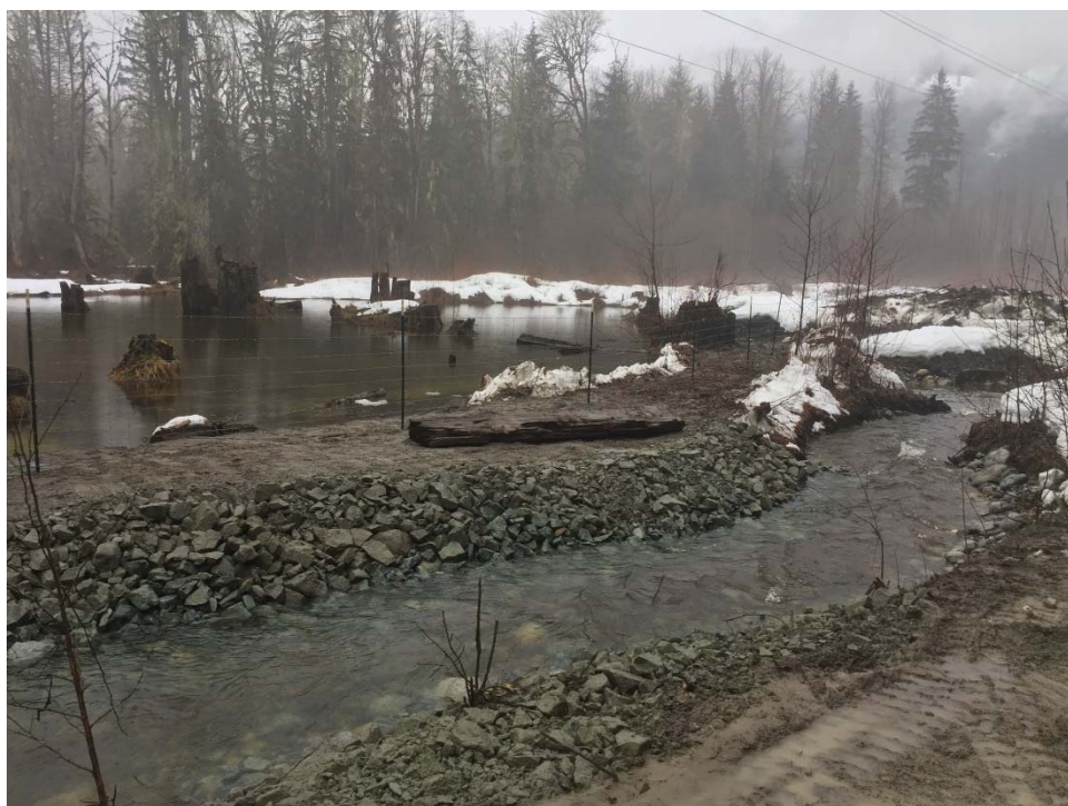
Fencing (photo taken March 20, 2017)
