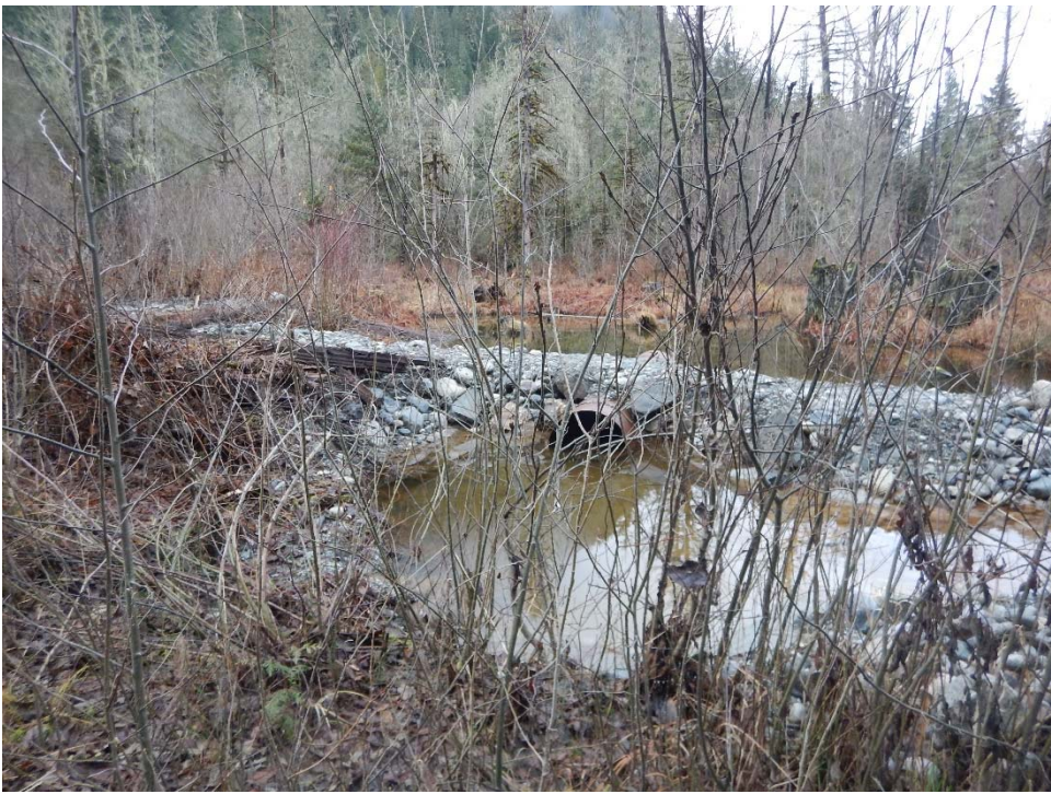
Facing north between “Culvert 1” and “Culvert 2”; note new connector culvert
