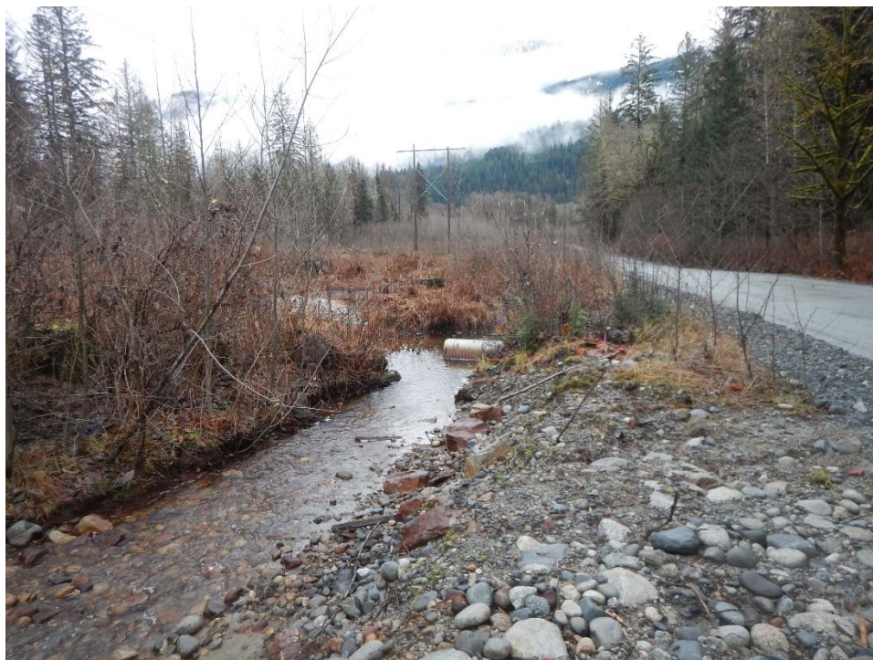
Facing east towards “Culvert 3”
