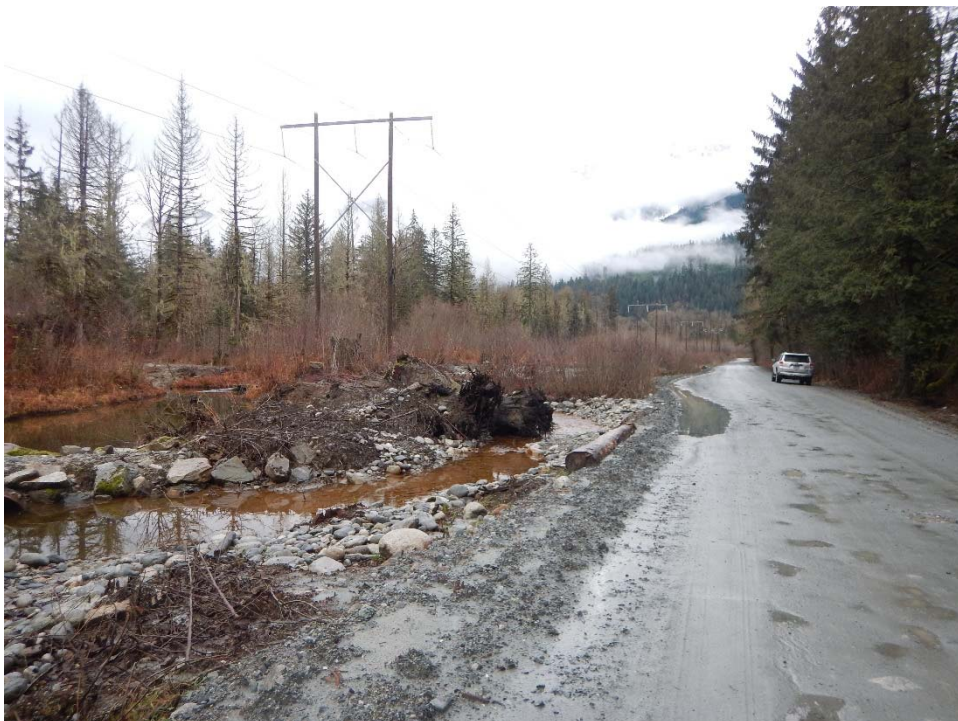
Facing east towards "Culvert 1"
