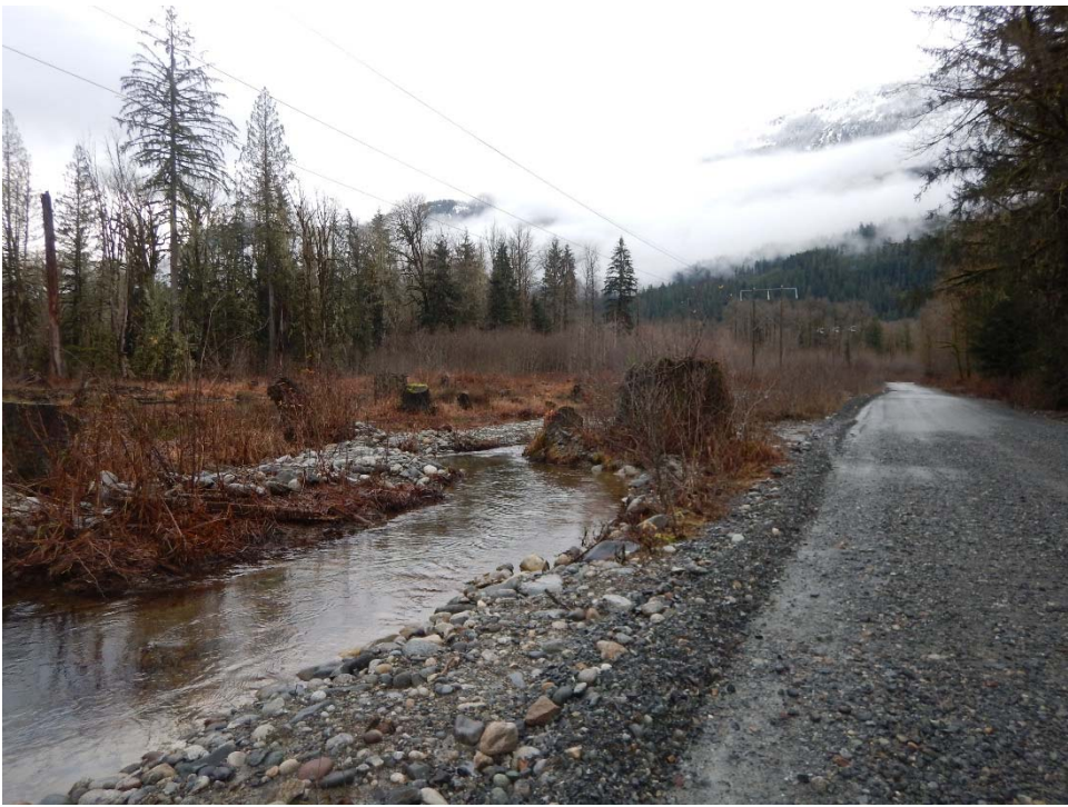
Facing east towards “Culvert 4”
