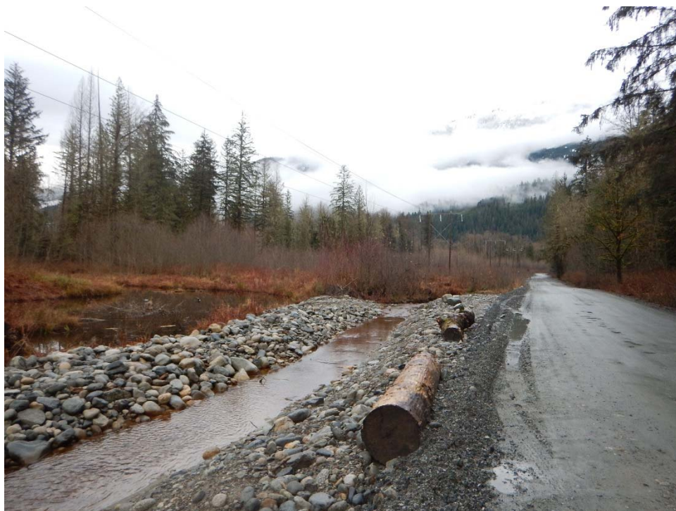
Facing east towards "Culvert 2"
