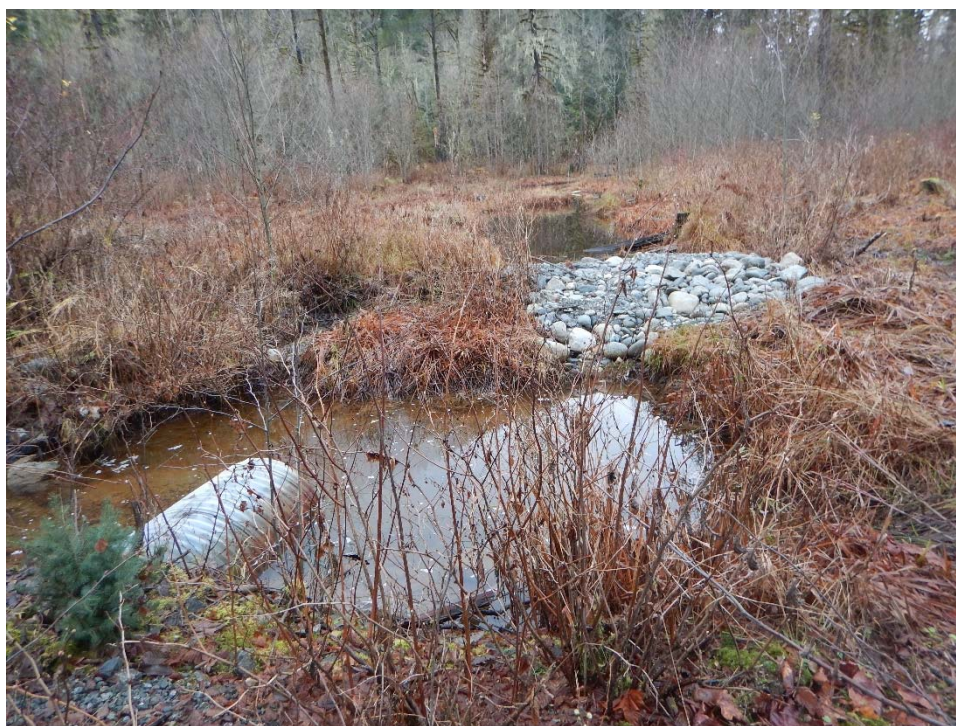
Site #6 “Culvert 2” – facing upstream, north of road; note gravel weir to maintain rearing habitat (top of photo)
