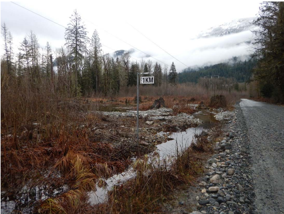
Facing east towards "Culvert 3"
