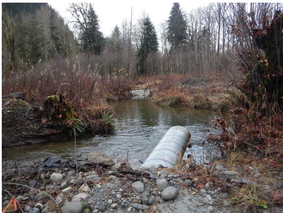
“Culvert 4” – facing upstream on north side of road
